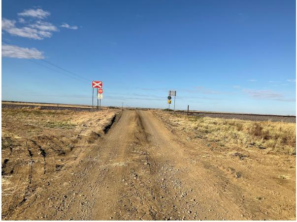
Figure 20: Barabon Terranburby Road – Steep ascent at Railway Crossing at approach (South of Flinders Highway)
