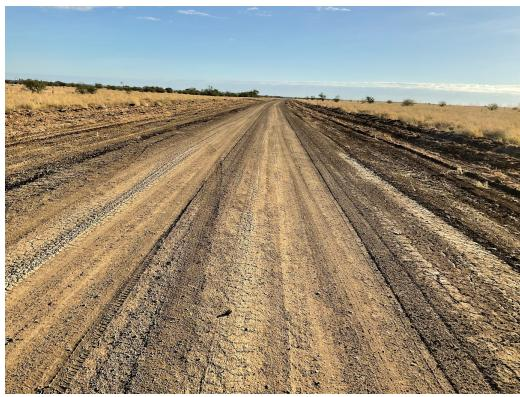
Figure 17: Marathon Stamford Road – Rutting, shoving and cracks
