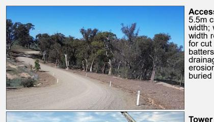
Access tracks: 5.5m crest width; wider toe width required for cut / fill batters; drainage and erosion control; buried cabling.
