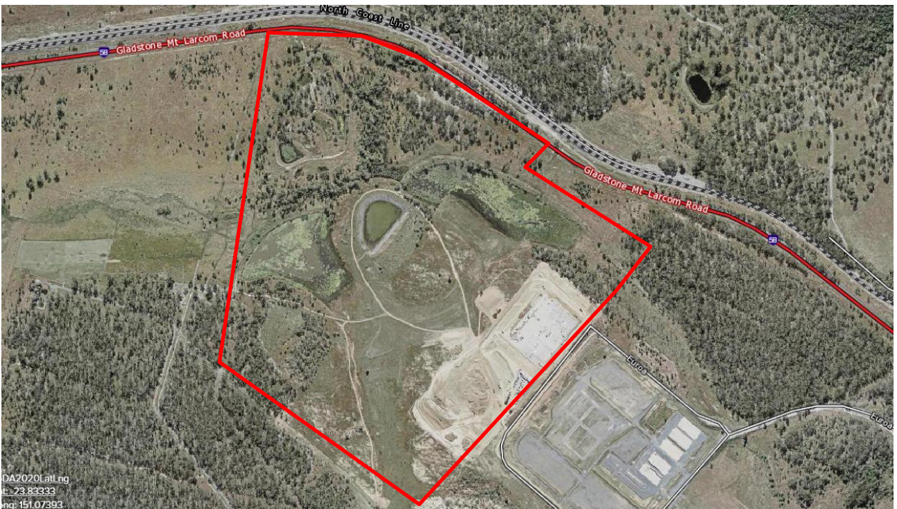
Figure 3-10 Existing vegetation screening the Site from Gladstone – Mt Larcom Road Source: QLD Globe
