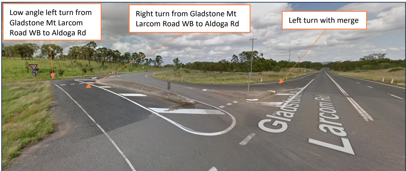
Figure 7: Gladstone Mt Larcom Road/Aldoga Road intersection (Source: Google Streetview, 2018)
