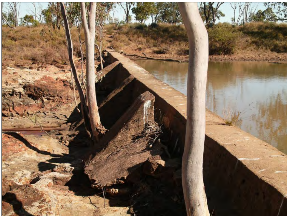
Figure 17: View south showing the largest Creek Farm Overshoot wall and buttresses
