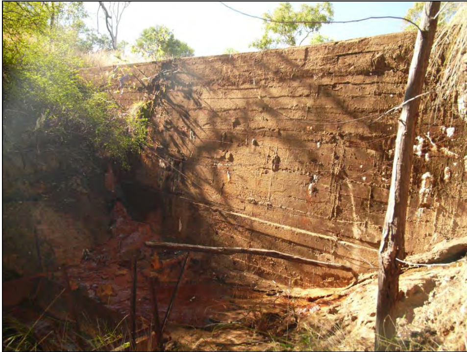
Figure 22: View south showing the dam face, with valve and trough at its base
