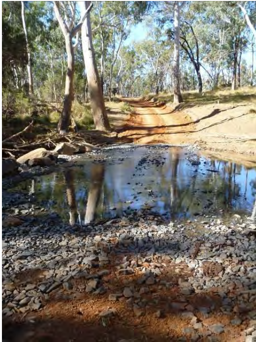
Figure 3-17: Constructed causeway at AC-1
