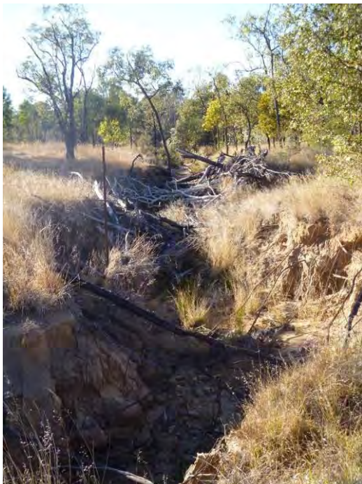
Figure 3-18: Severe gully head erosion associated with a washed out farm track in upper Sapling Creek
