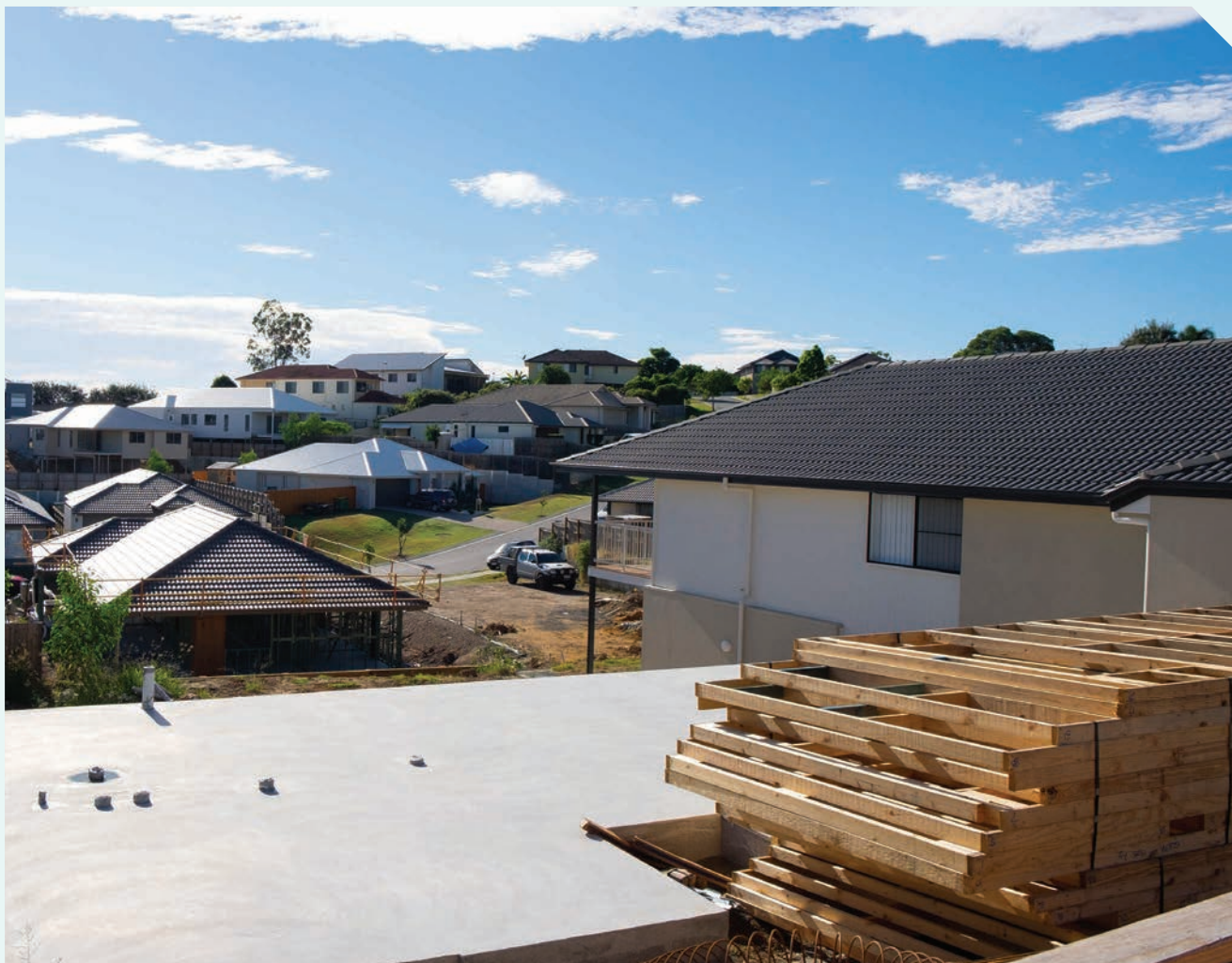
Growth area house under construction
