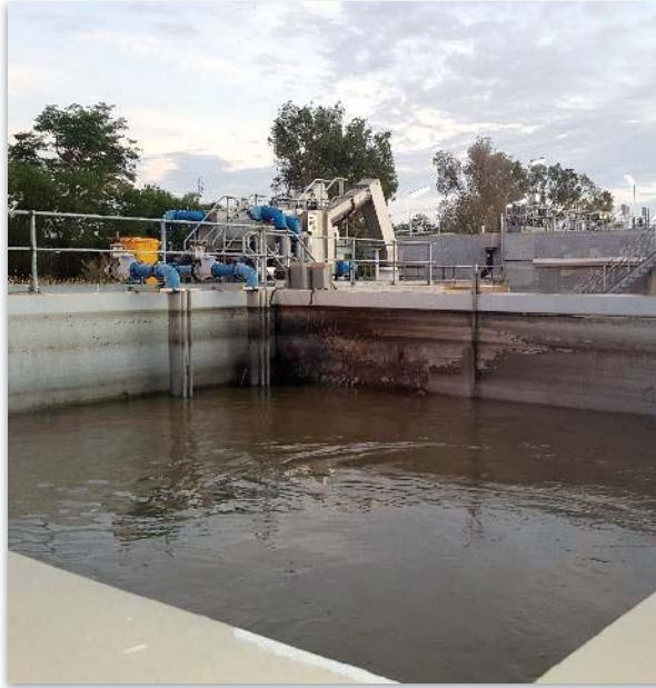
Figure 3 – Flow Balance Tank and Submersible Pumps
