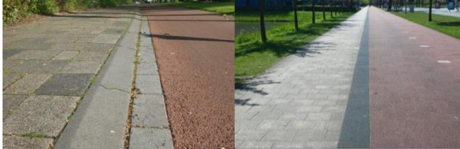
Figure 8-28 Diagonal edge and no edge treatment for pedestrian path/cycle track transition
