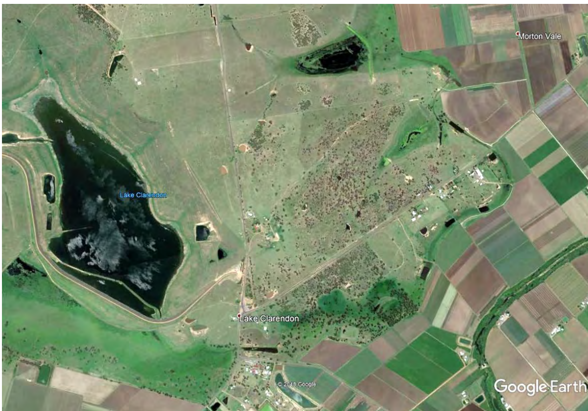
Figure 8.2 Example of water storages scattered throughout the Lockyer Creek catchment
