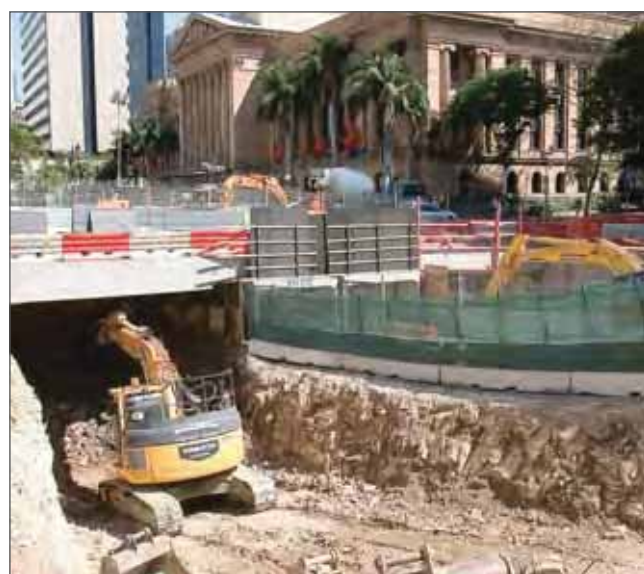
Construction, King George Square Busway
