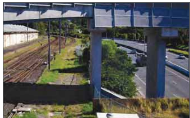
Exhibition Loop, Inner Northern Busway and Inner City Bypass
