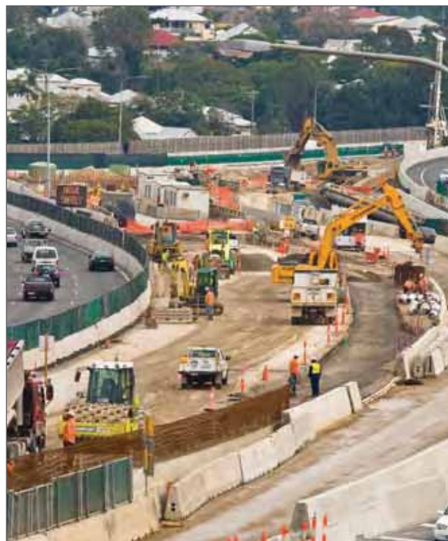
M3 surface works, Clem Jones tunnel Photo courtesy of Leighton Contractors
