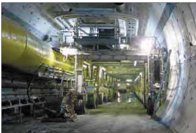
Tunnel boring machine, Clem Jones tunnel
