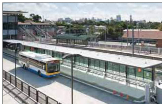
Existing bus – rail interchange, Boggo Road
