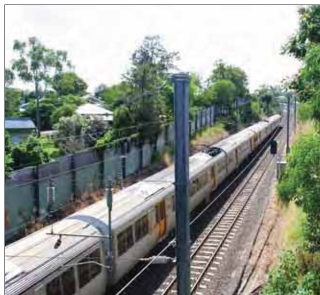
Rail corridor noise attenuation, Fairfield
