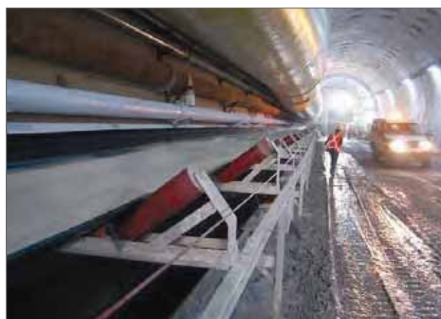
Construction, Clem Jones tunnel
