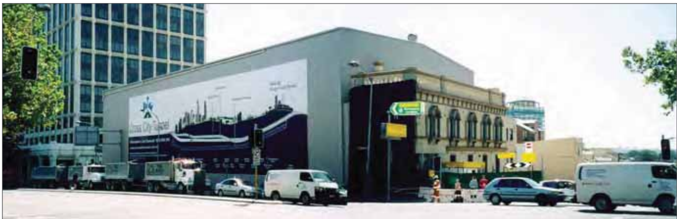
Worksite Cross City Tunnel, Williams Street, Sydney
