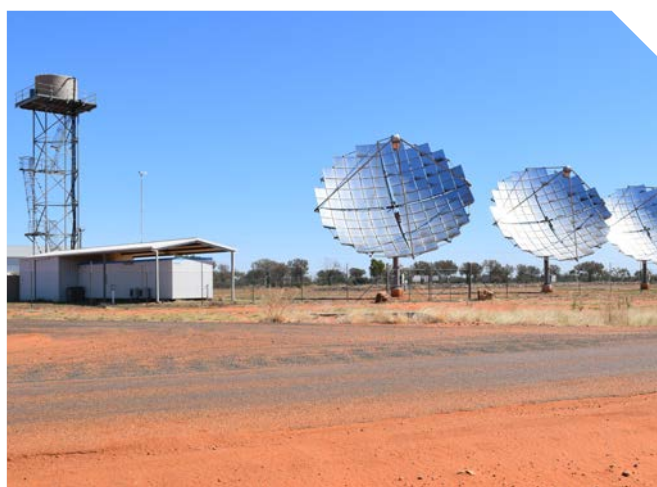
Ergon Energy's Windorah Solar Farm, uses five concentrated solar dishes (Source: DSDILGP)
