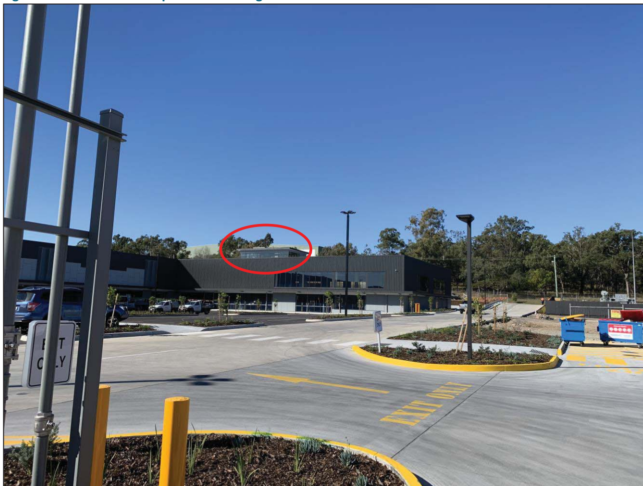
Figure 16: Enclosed Roof Space on Building 1
