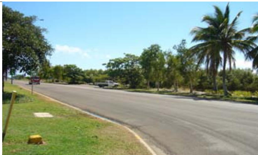
Existing Ross River foreshore and Benwell Road
