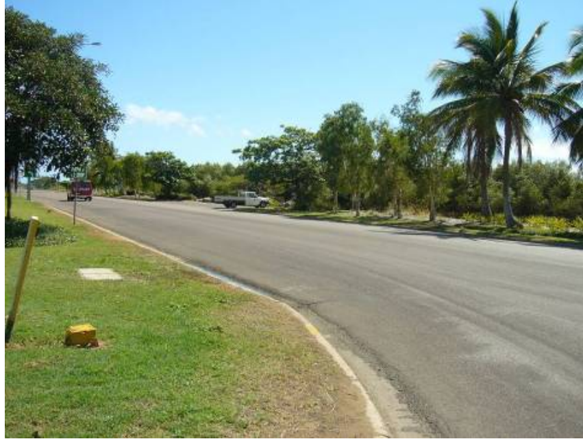
Existing Ross River foreshore and Benwell Road
