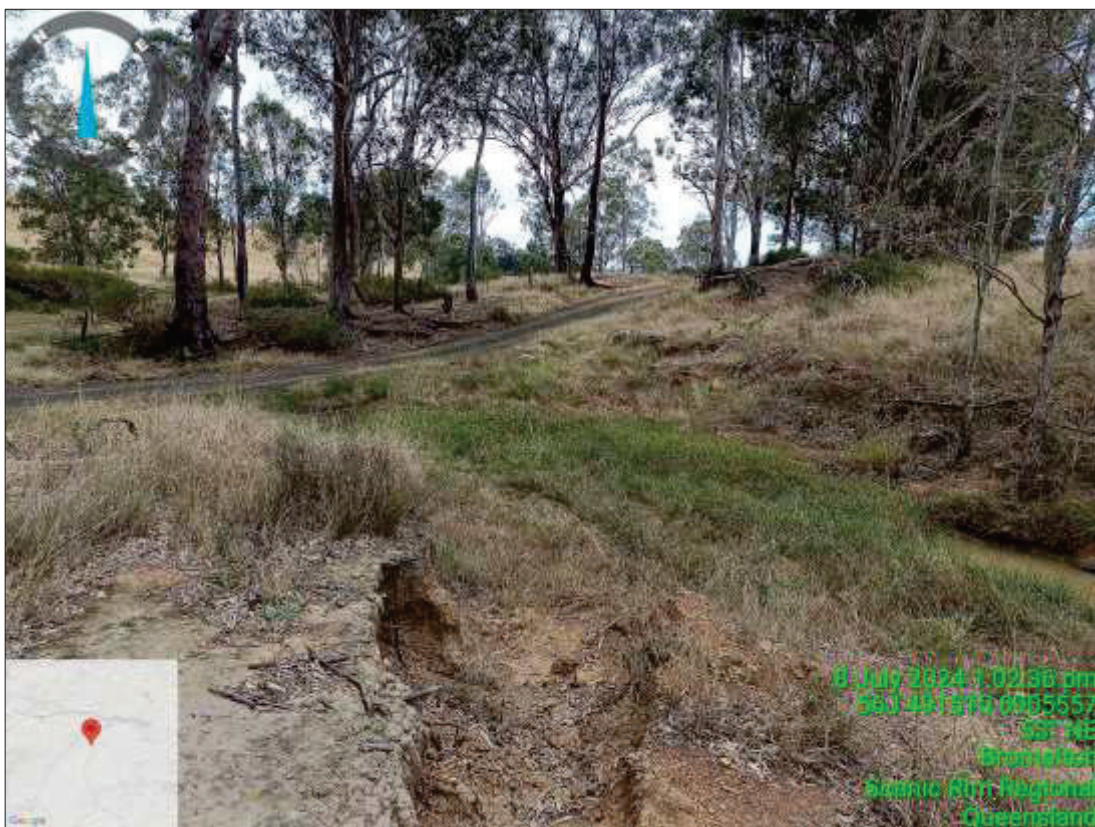
Photograph 6: Creek at north of the site, showing evidence of erosion
