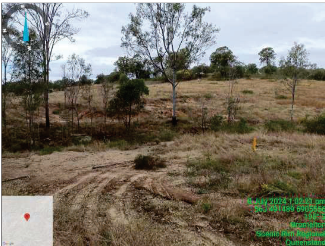
Photograph 4: From northern side of the site, looking east, also showing creek with scour erosion
