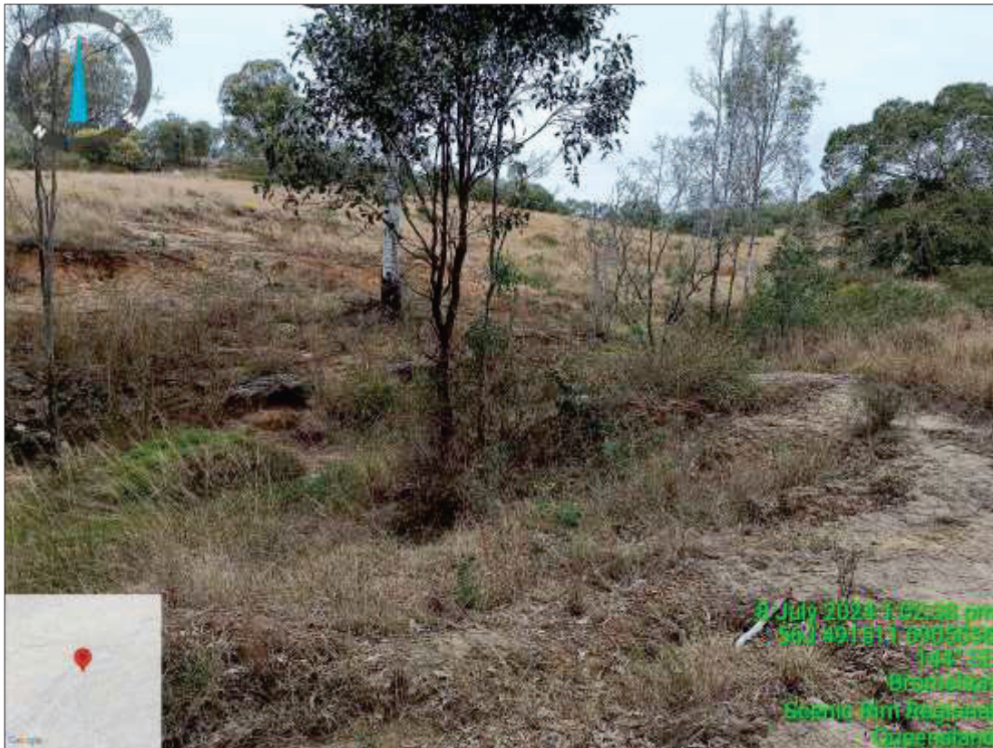
Photograph 5: Creek at north of the site, showing evidence of erosion
