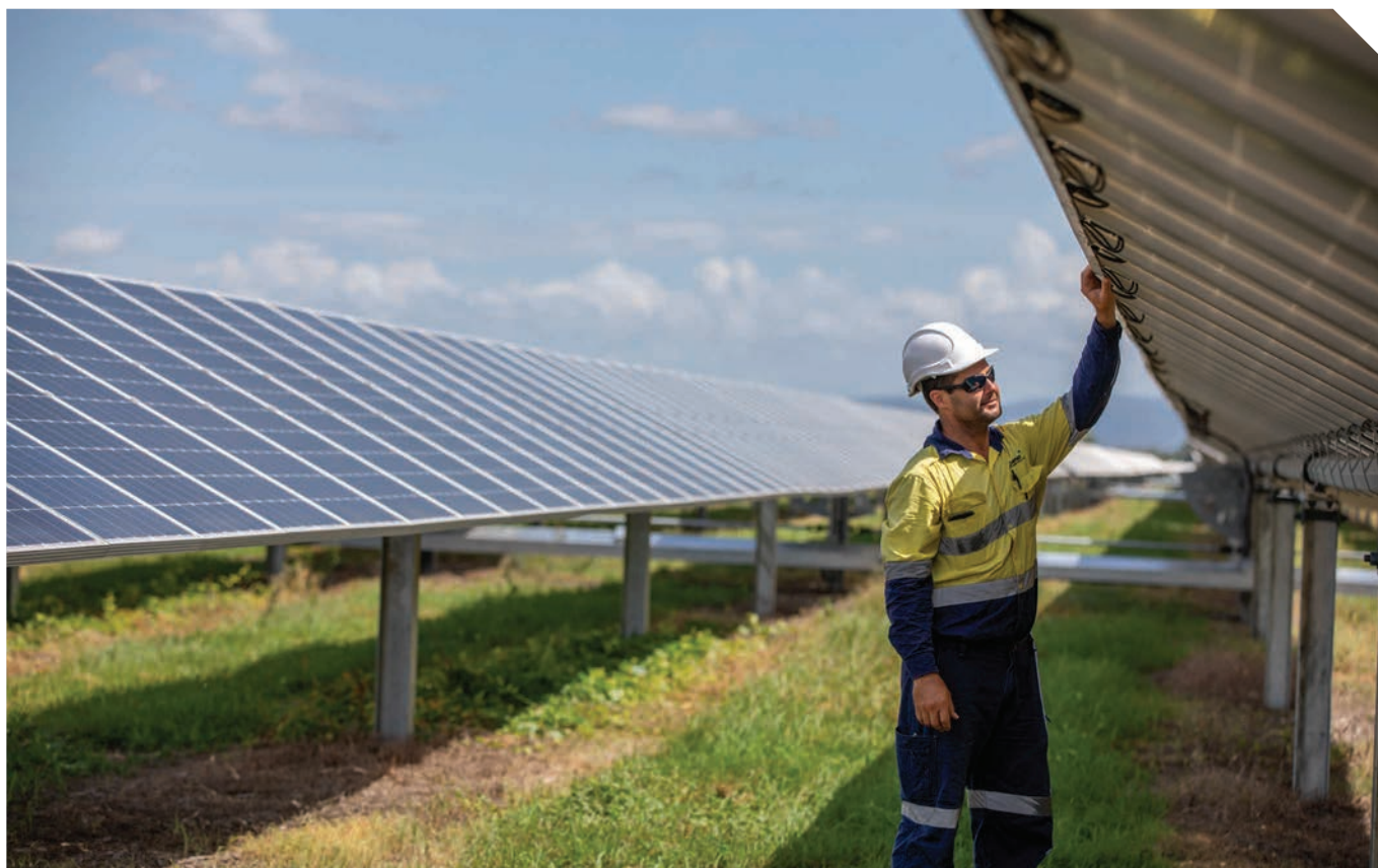
Ross River Solar Farm, Townsville
