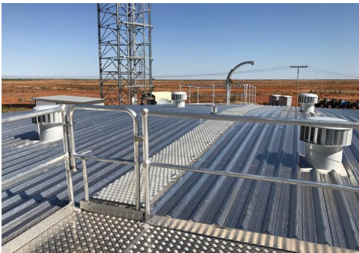
Above: the new roof in place on the Boulia Reservoir.
