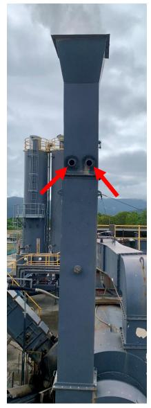
Figure 1: Asphalt Plant Chimney Stack Sampling Locations
