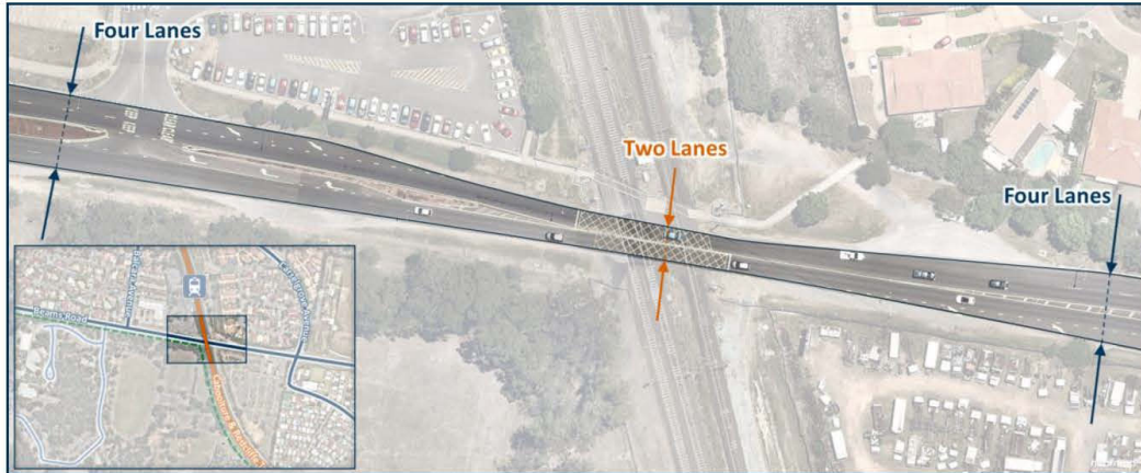
Figure 2-9 Beams Road Open Level Rail Crossing
