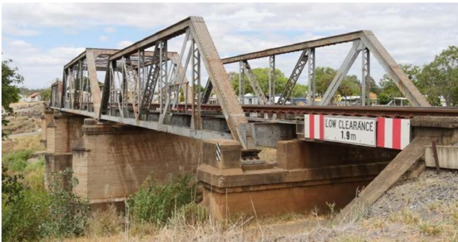
Photograph 6.6 Lockyer Creek Bridge (H2C-19-H06)
