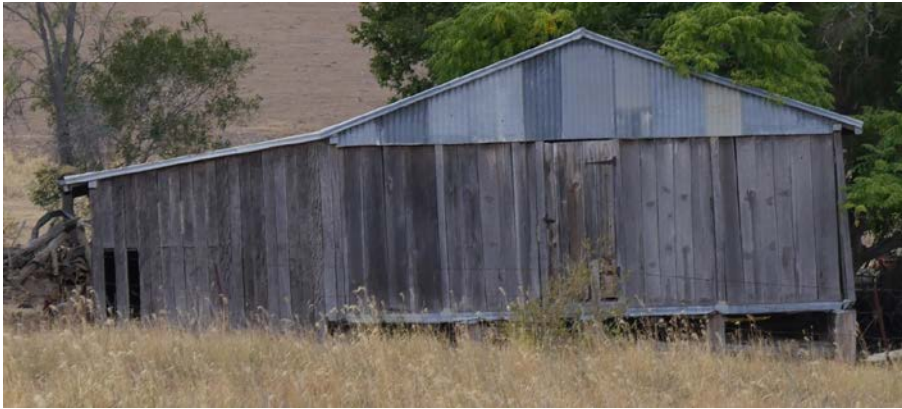
Photograph 6.44 Outbuilding with timber slabs (H2C-19-H28)
