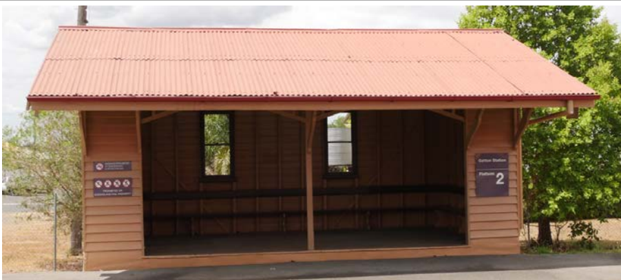
Photograph 6.9 Platform shelter (front) (H2C-19-H07)
