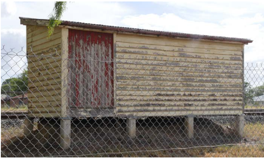
Photograph 6.31 Goods Shed (H2C-19-H19)
