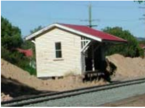
Photograph 6.36 Platform shelter at Forest Hill Railway Station (Buchanan Architects 2002)
