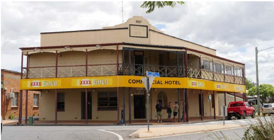
Photograph 6.17 Commercial Hotel (H2C-19-H11)
