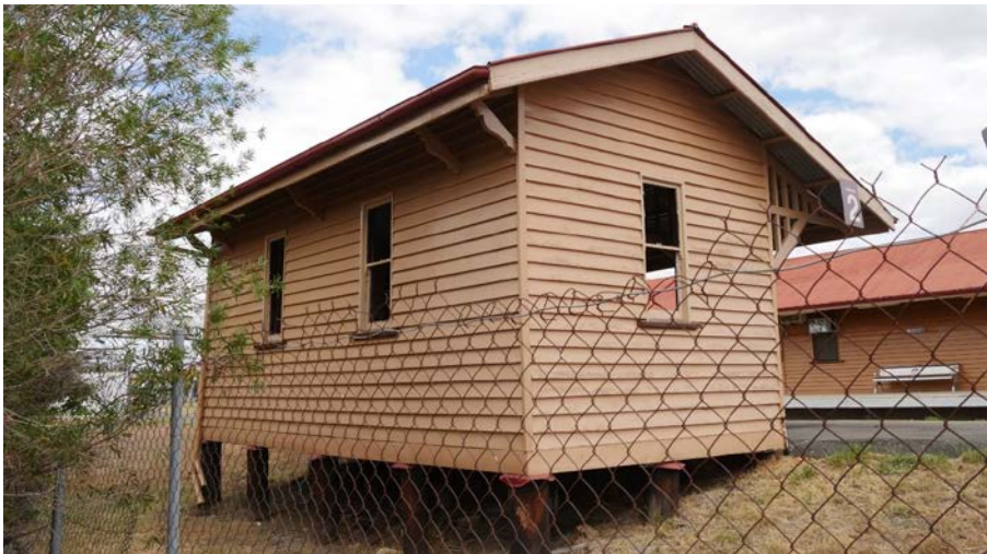
Photograph 6.8 Platform shelter (rear) (H2C-19-H07)
