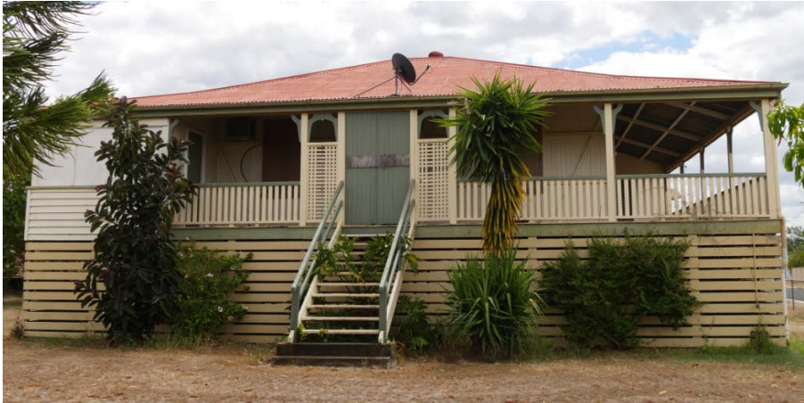
Photograph 6.14 Gatton Station Master's Residence (H2C-19-H08)
