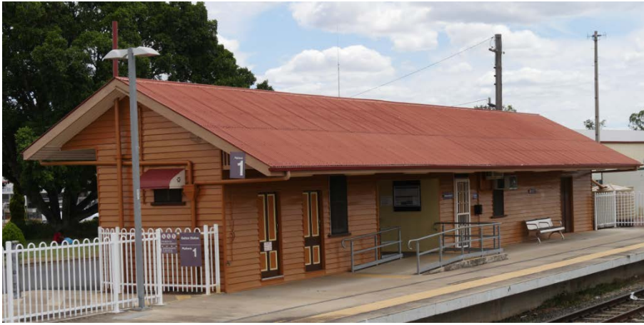
Photograph 6.12 Passenger station (rear) (H2C-19-H07)
