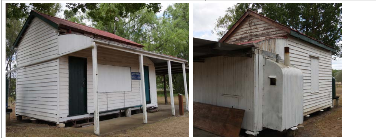
Photograph 6.53 Crew Quarters (former) (H2C-19-H35)
