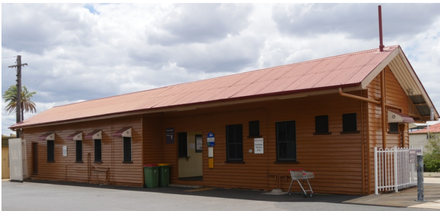
Photograph 6.11 Passenger station (front) (H2C-19-H07)
