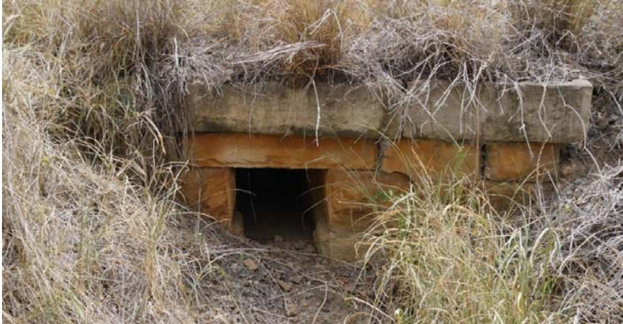
Photograph 6.1 Sandstone culvert (H2C-19-H01)
