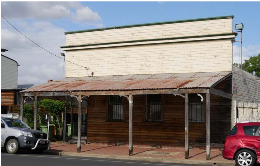
Photograph 6.39 National Bank (former) (H2C-19-H24)
