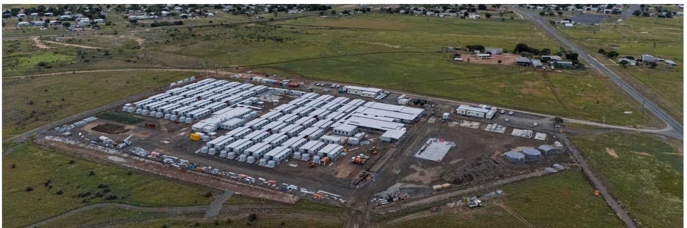
Hughenden workers accommodation - Powerlink
