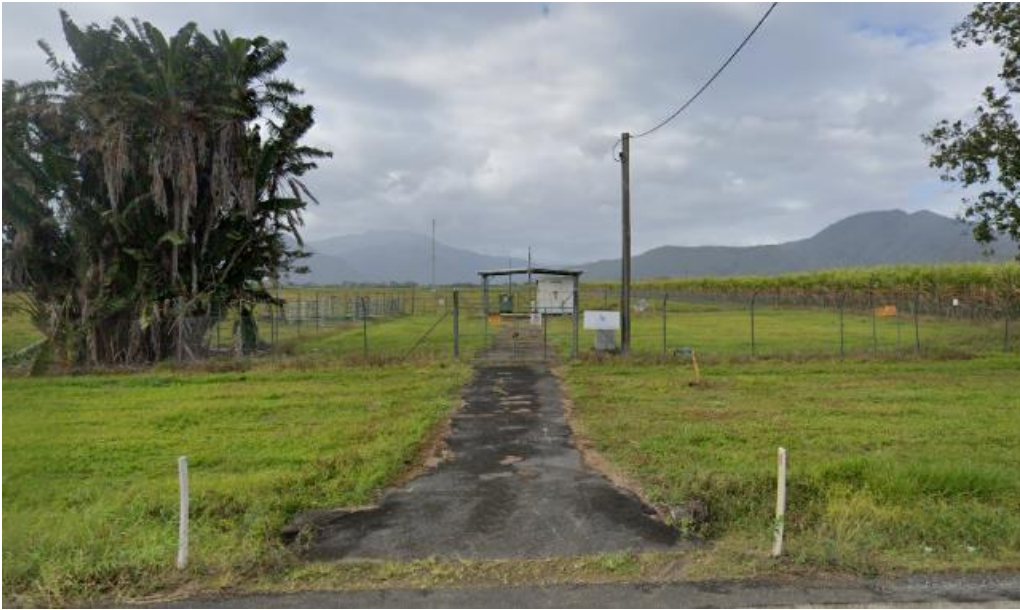
Figure 13 Radio Shed at 94 Warner Road (source google)
