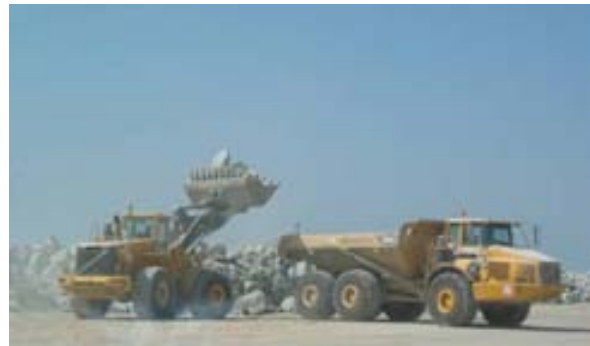
Loader rehandling armour to offroad dump truck
