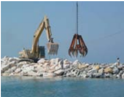
Excavator and grab barge placing rock offshore
