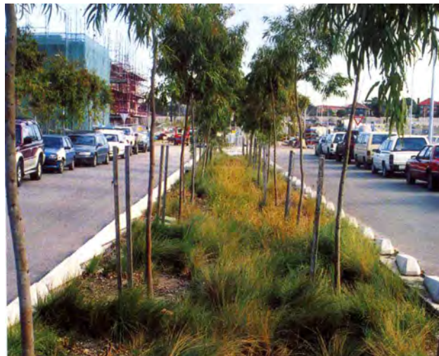
Vegetated bioretention swale
