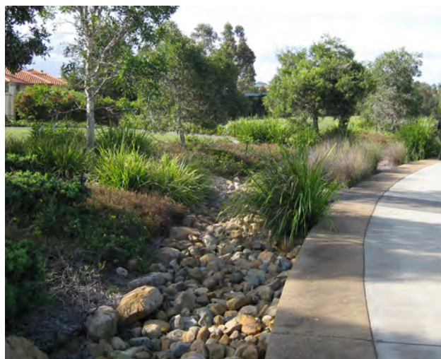
Rock-lined and vegetated bioretention swale
