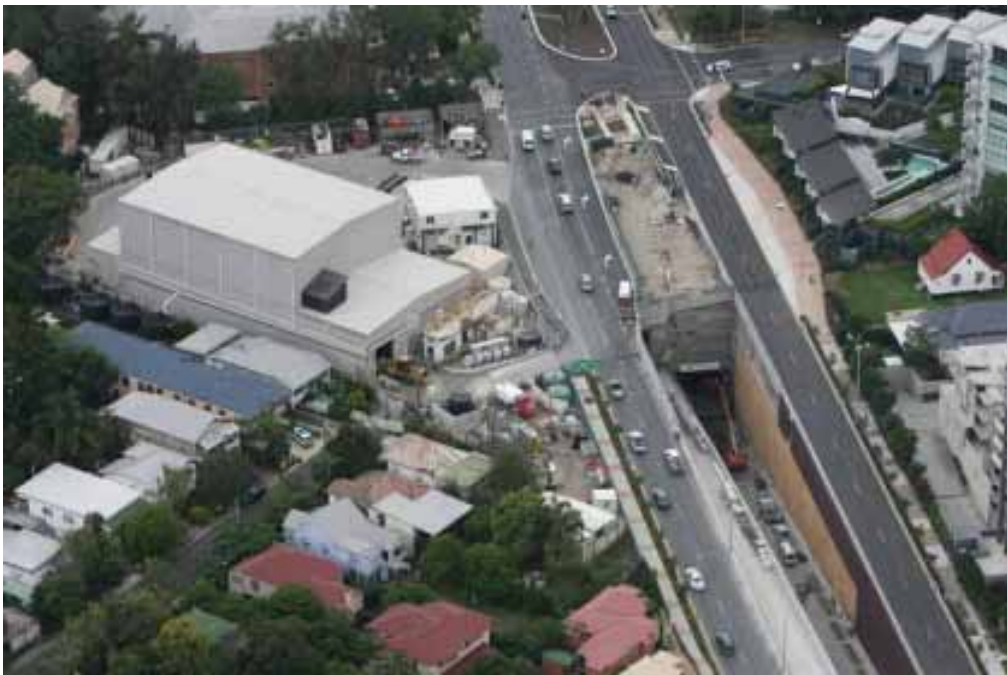
Figure 4 – Shaftston Acoustic Shed
