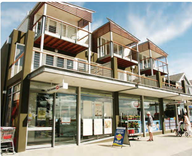
Figure 3: Visually interesting facades
