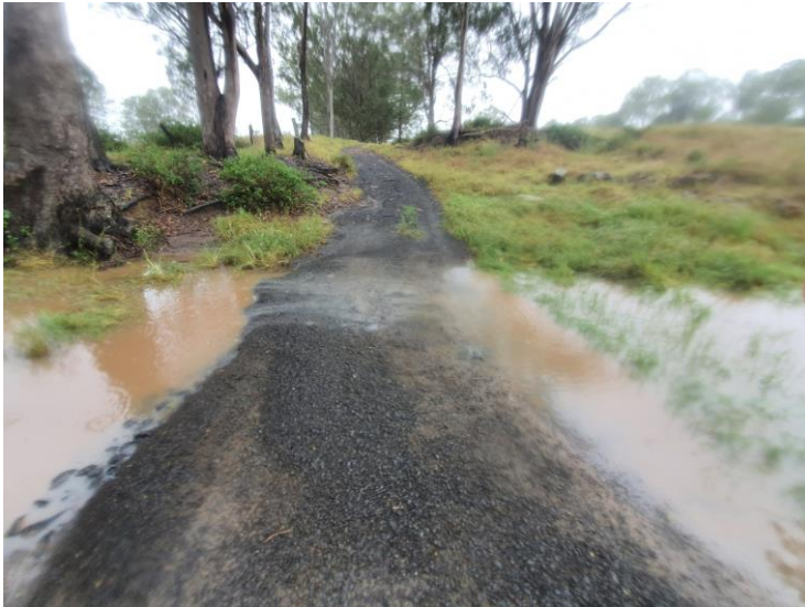
Figure 4.1 Waterway crossing of Allan Creek tributary 3
