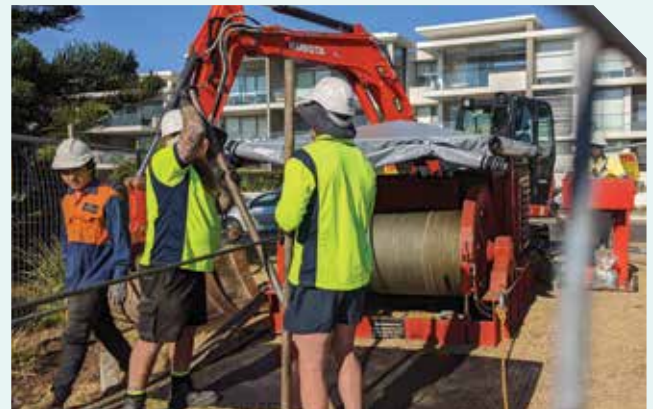
Laying cable (Source: Queensland Capacity Network Pty Ltd, trading as QCN Fibre)
