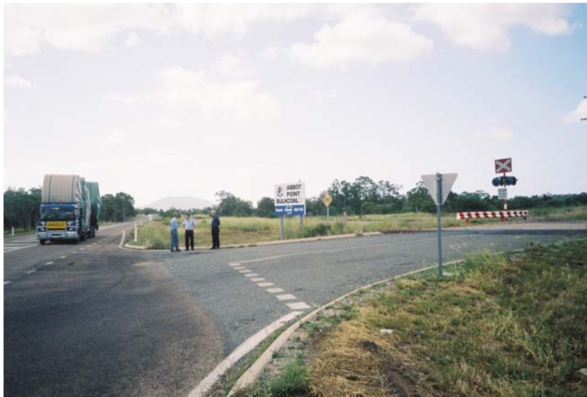
Photo 4a: Bruce Highway – Abbot Point Access Road intersection, looking north
