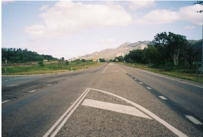
Photo 4b: Bruce Highway – Abbot Point Access Road intersection, looking south
