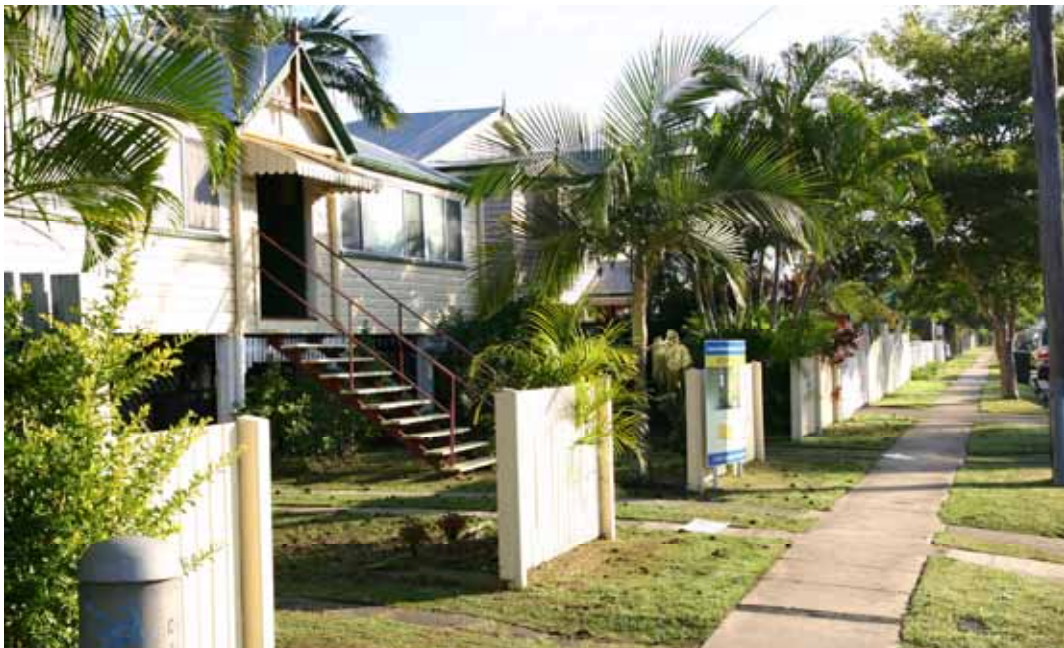
Photo 2-2: Residential Dwellings, Kent Road
