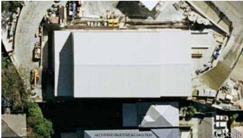
Photo 5-7: Aerial View of Acoustic Shed Located at Shaftson Avenue (CLEM7)
