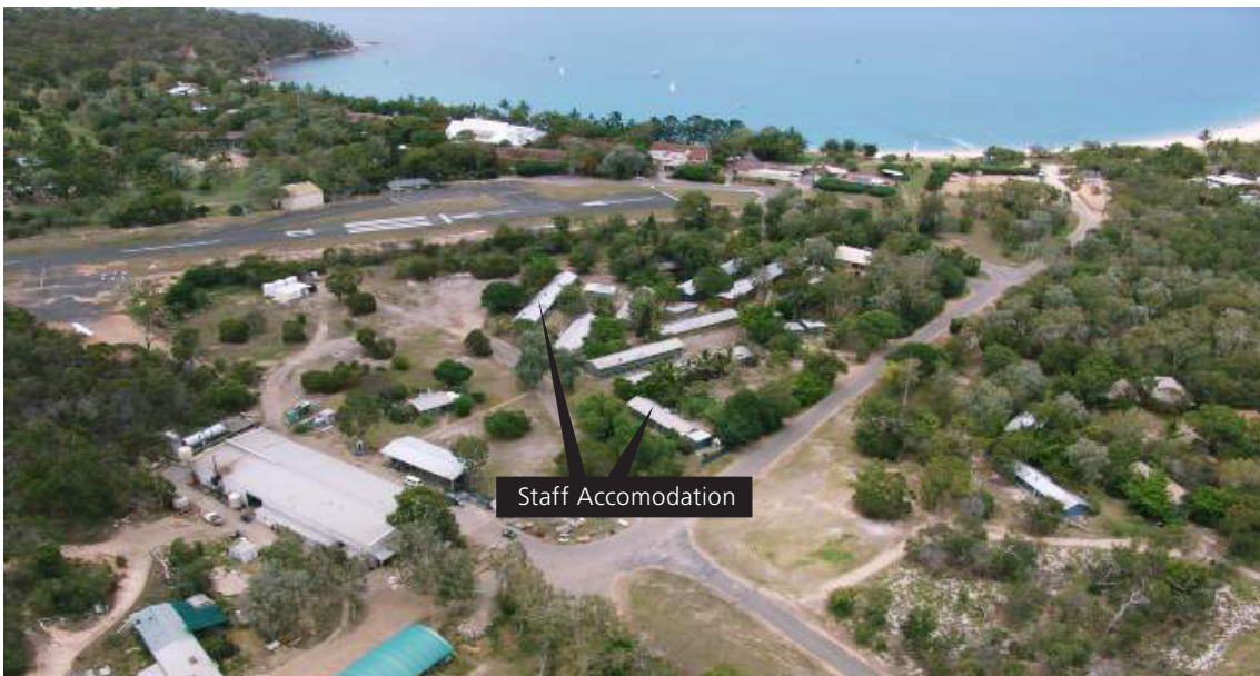
Photograph ES.7 AERIAL VIEW OF FORMER RESORT FACILITIES (STAFF ACCOMMODATION)
