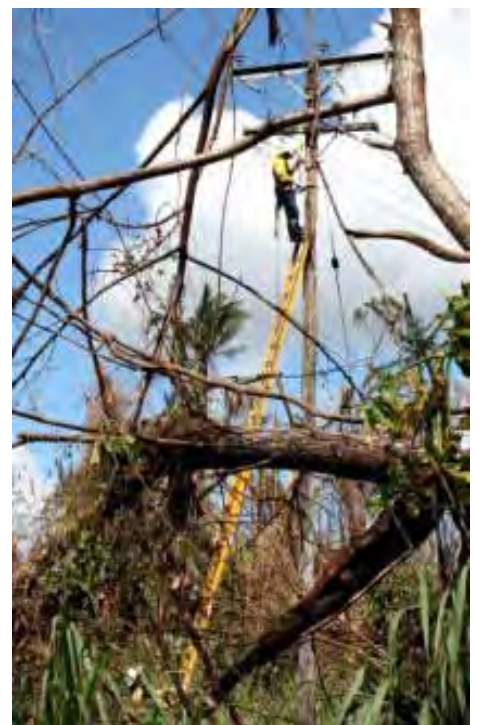
Photo 3 courtesy of Ergon Energy – Repairing the network in Tully
