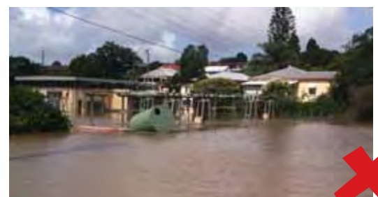
Photo 1: Example of an older, non-resilient substation design
