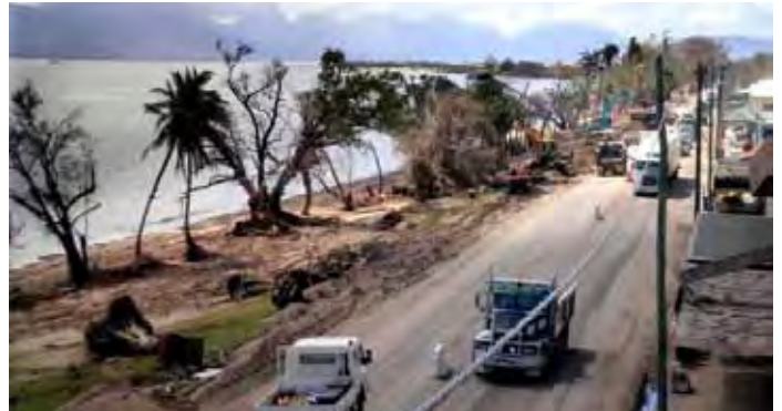
Photo 2: Courtesy of Ergon Energy - Highway through Cardwell post Cyclone Yasi, featuring overhead bundled cable
