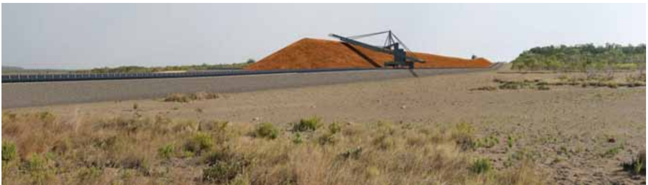
Figure 3-13: Proposed bauxite stockpile showing conveyor, bauxite stockpile and stacker-reclaimer.
