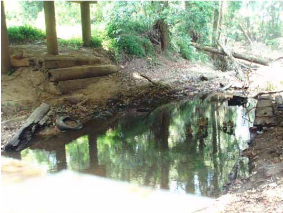
Plate 10: North Maroochy River adjacent and downstream of the crossing point (facing north east). Northern bank with little or no riparian vegetation under road bridge, and evidence of bank erosion.
