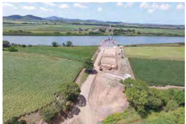
Mackay Ring Road Pioneer River bridge (image courtesy of CPB Contractors)
