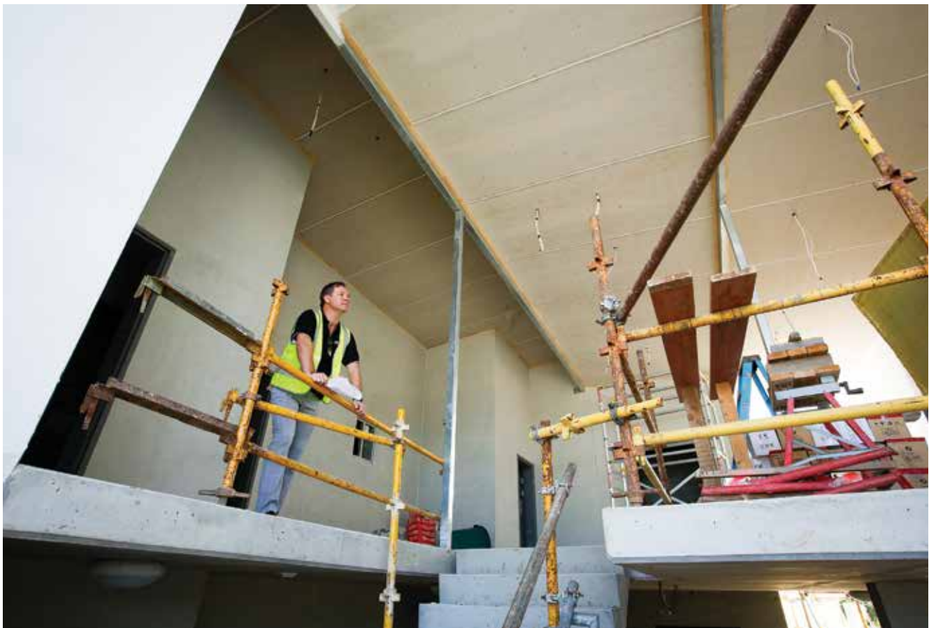
Social housing construction
