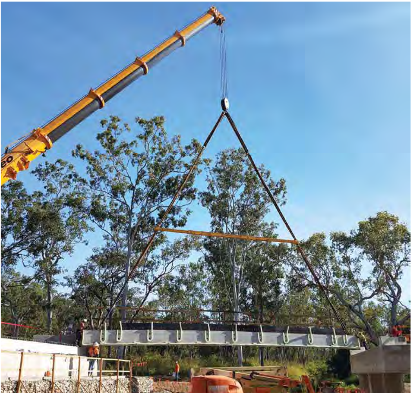
Peak Downs Highway structure replacement
