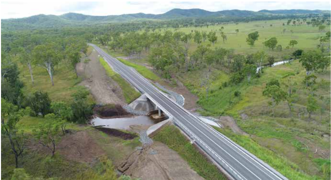
Dawson Highway (Gladstone – Biloela) timber bridge replacement package
