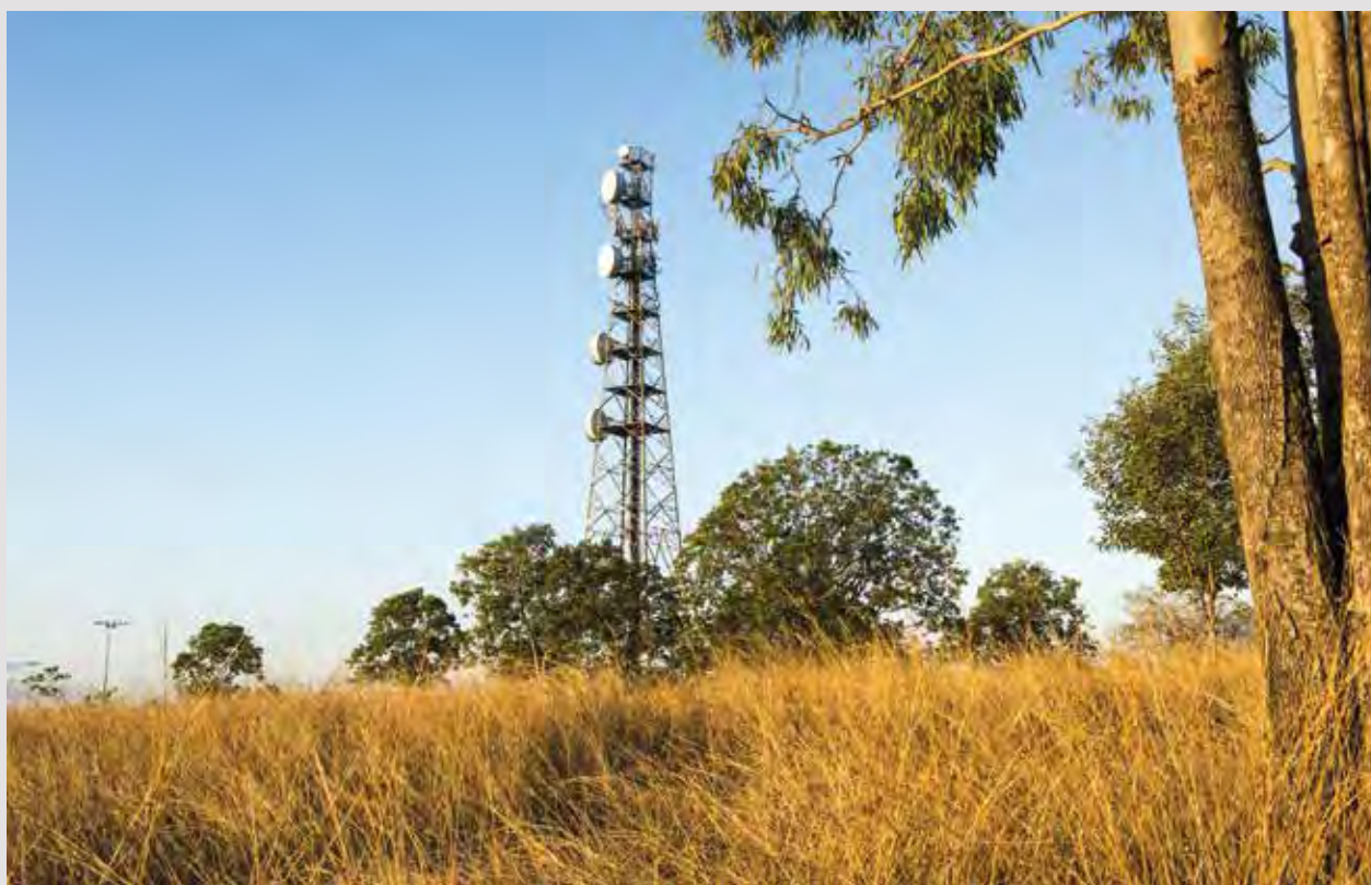
Mobile phone tower, Queensland
