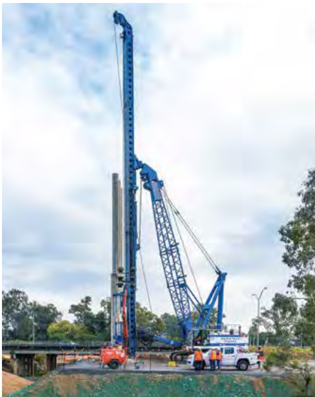
Bridge piling works underway, Ipswich Motorway Upgrade – Rocklea to Darra stage 1
