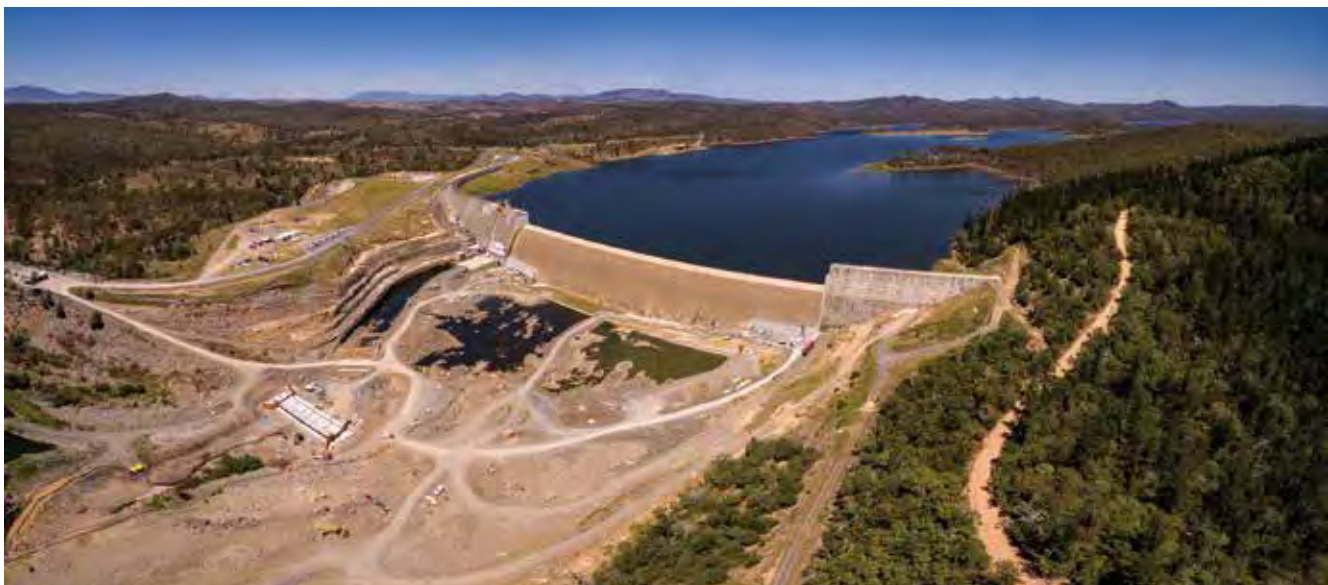
Paradise Dam, Wide Bay–Burnett region
