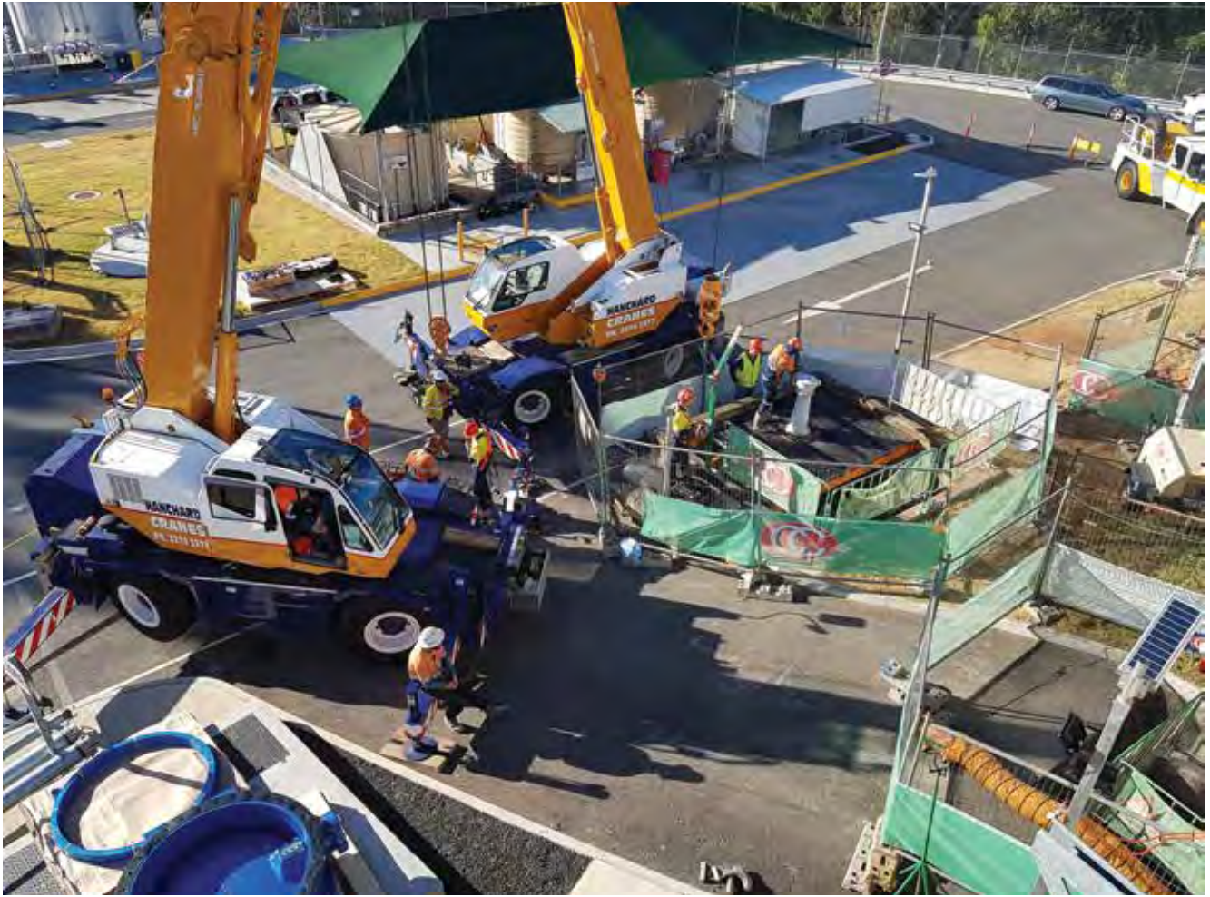
Mount Crosby East Bank Water Treatment Plant
