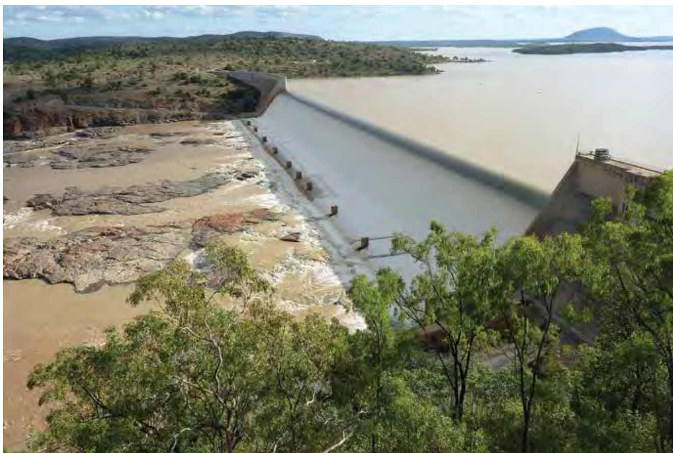
Burdekin Falls Dam improvement
