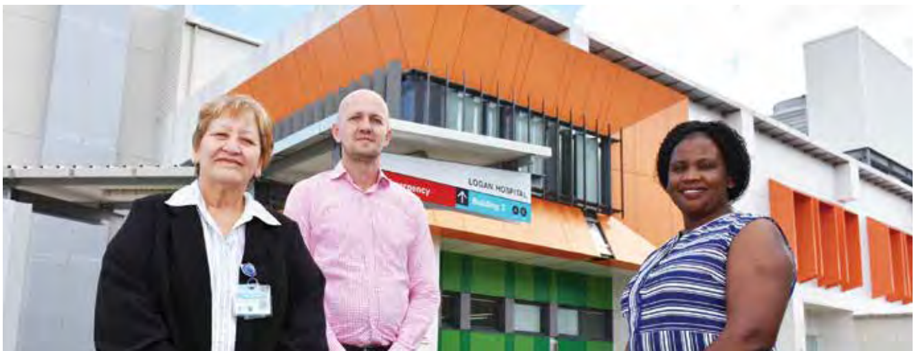
Logan Hospital expansion is in the detailed business case phase of the Building Queensland Pipeline
