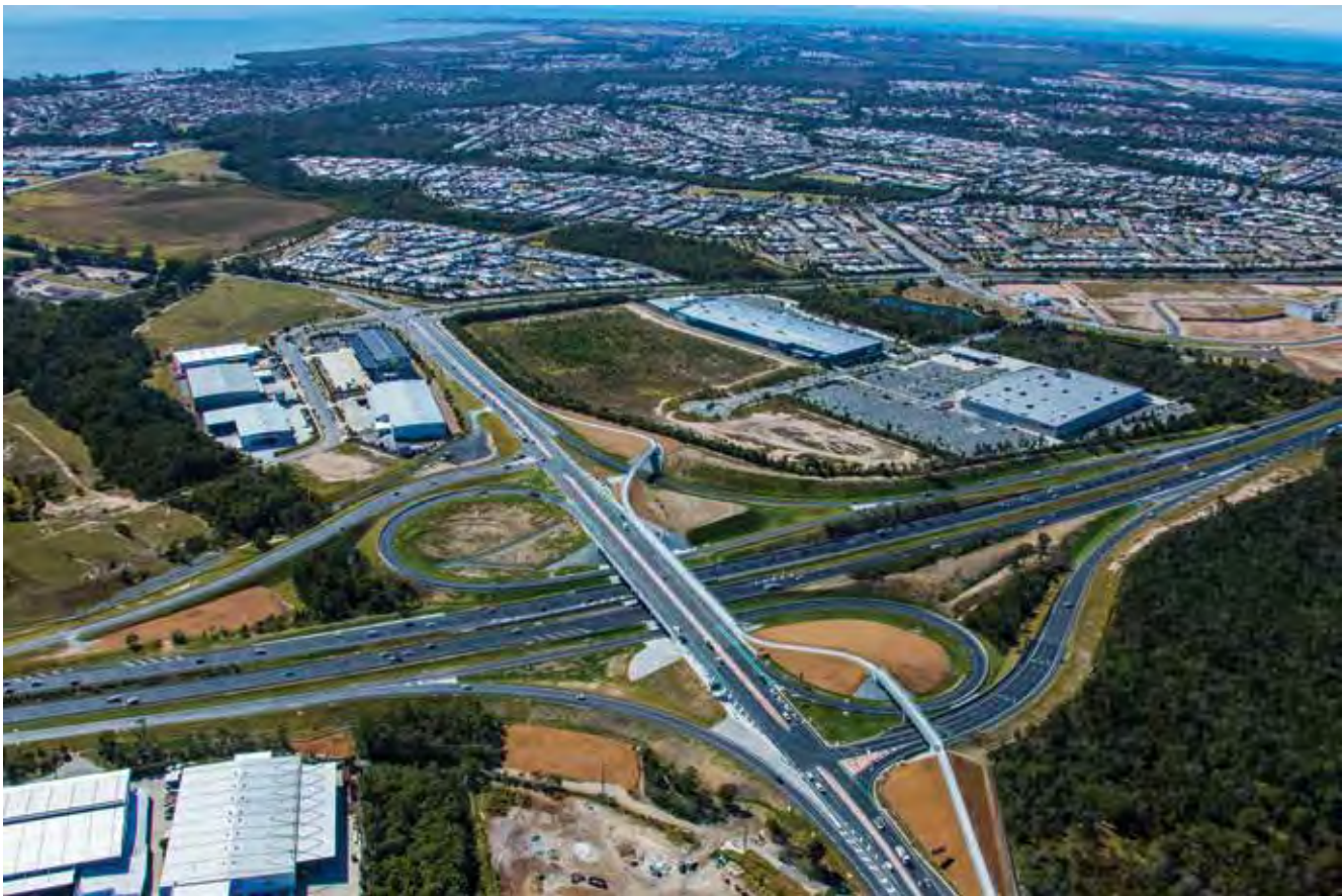
Boundary Road Interchange, Bruce Highway, Narangba
