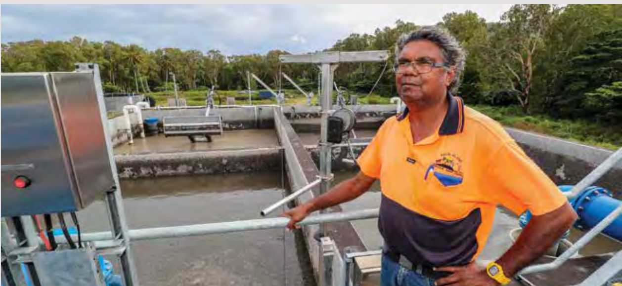
New water treatment plant, Palm Island
