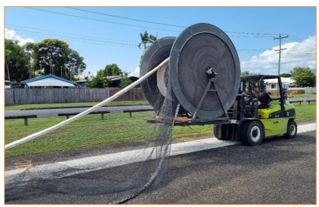
Figure 6: Net being rolled up on the hardstand. Source: Uninet
