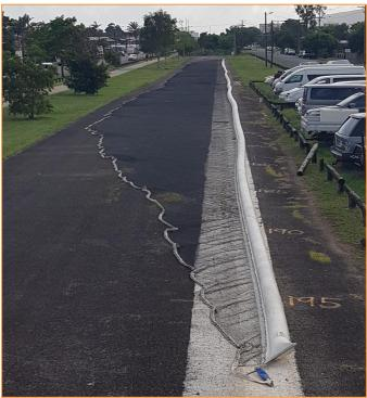
Figure 5: Net set out for inspection. Source: Uninet
