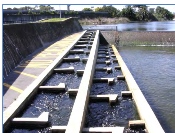
Figure 28 – Example of a Vertical-Slot Fishway
