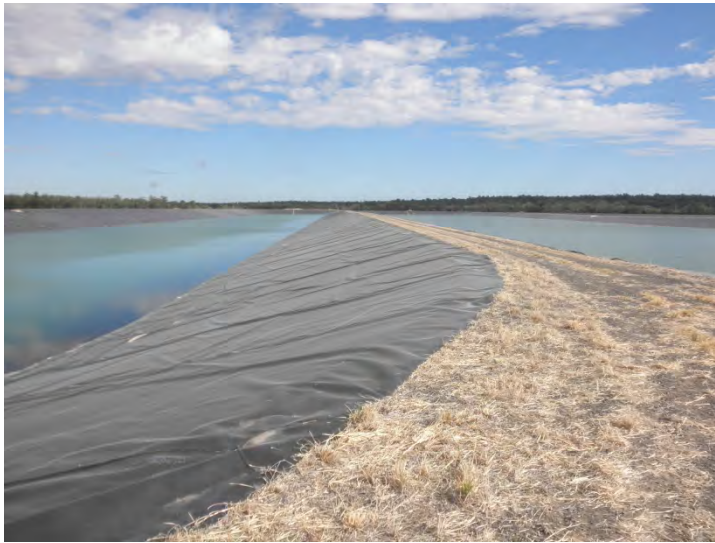
Figure 14 – Example of Large HDPE lined Storages
