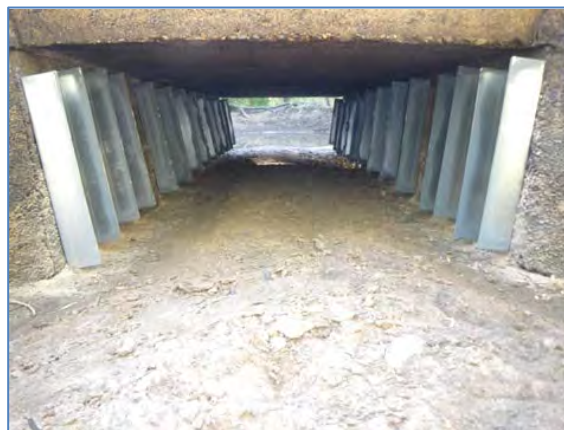
Figure 27 – Example of a Culvert Fishway with side baffles.
