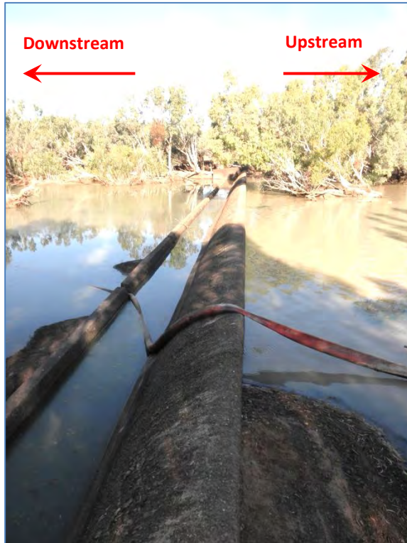
Figure 2 – Ogee Crest Area of Glenore Weir viewed towards Right Abutment
