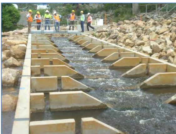
Figure 26 – Example of a Trapezoidal Weir Fishway.
