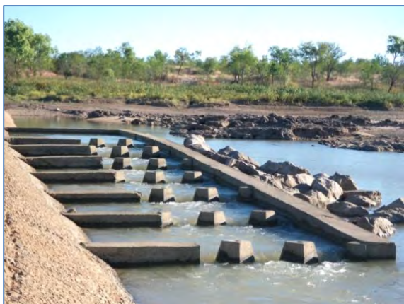
Figure 25 – Example of a cone Fishway on Flinders River
