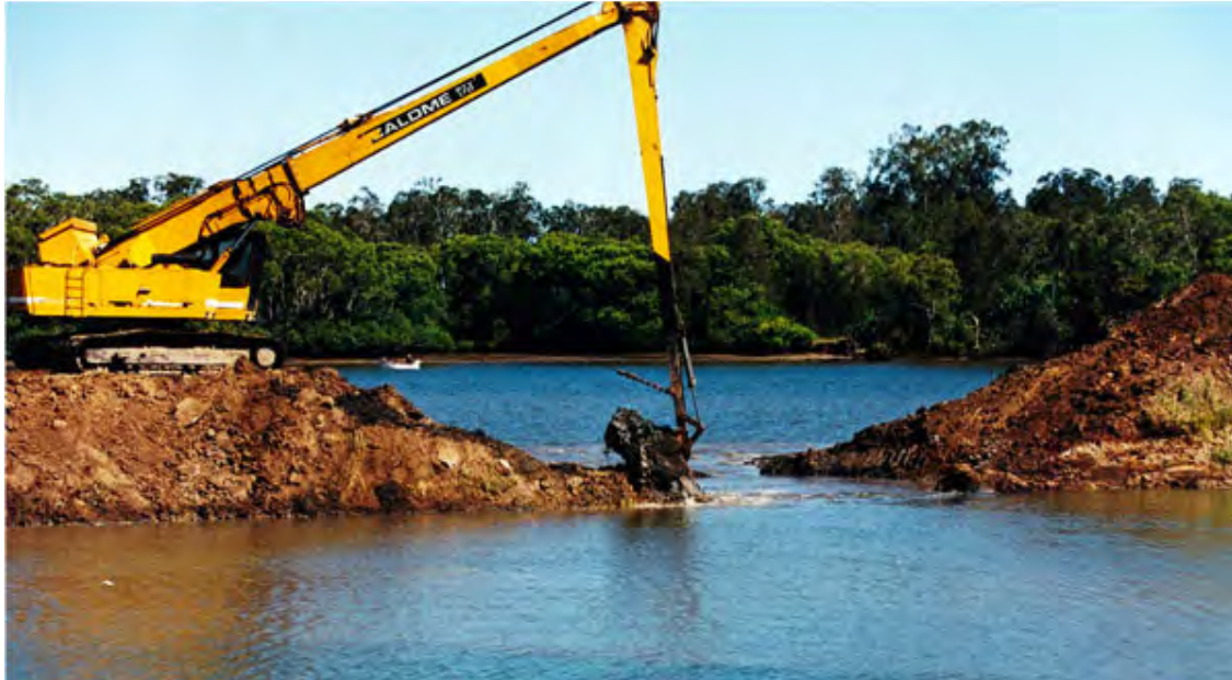
Figure 5.10 Dredging the entrance to the GCMP
