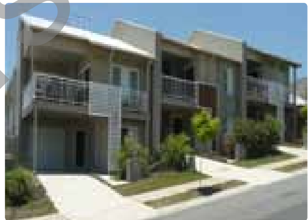
Dividing walls of terrace houses act as retaining walls to accommodate the slope of the land
