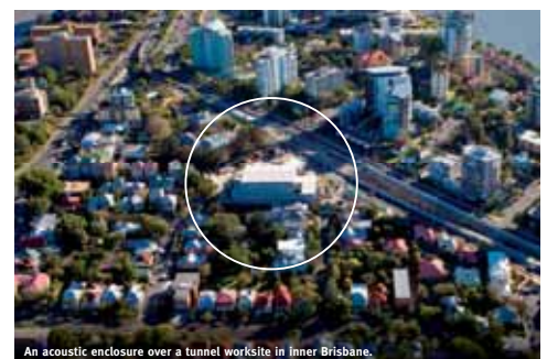
An acoustic enclosure over a tunnel worksite in inner Brisbane.
