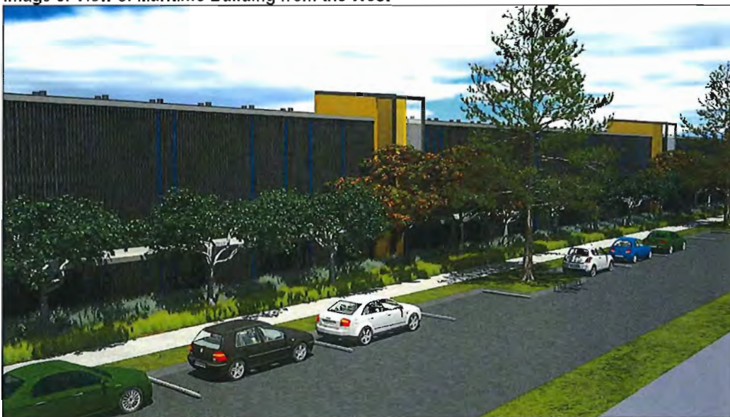
Image 6: View of Maritimo Building from the West
