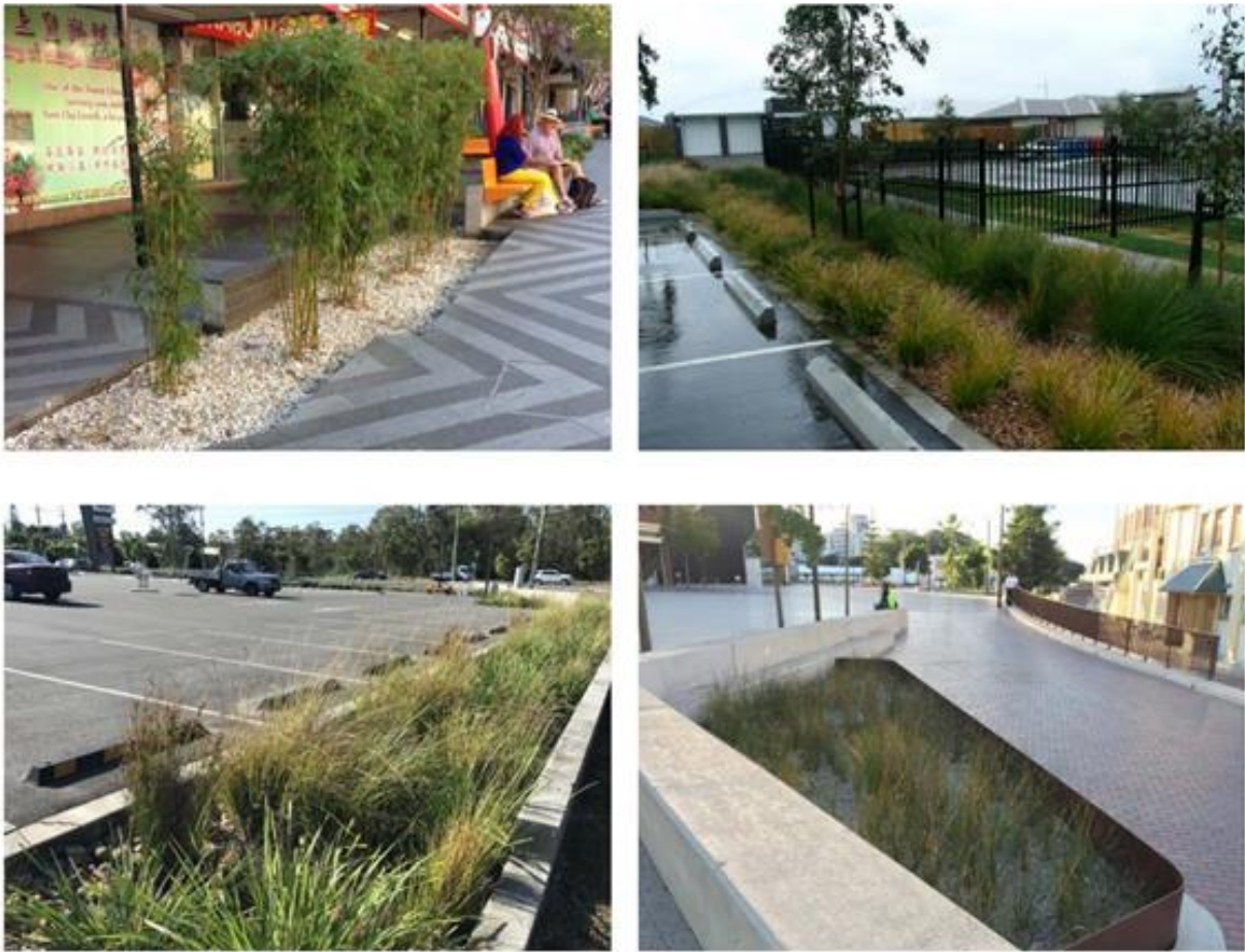
Figure 6-11 Bioretention basins and rain gardens
