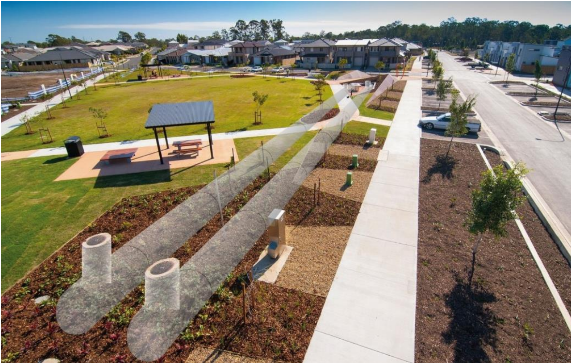
Figure 6-9: Stormwater Harvesting, Fitzgibbon Chase, Brisbane
