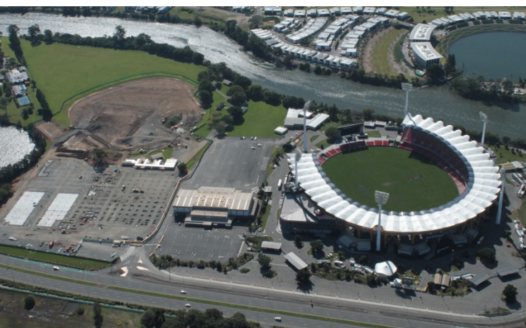
Aerial view of the Carrara Sports and Leisure Centre construction site
