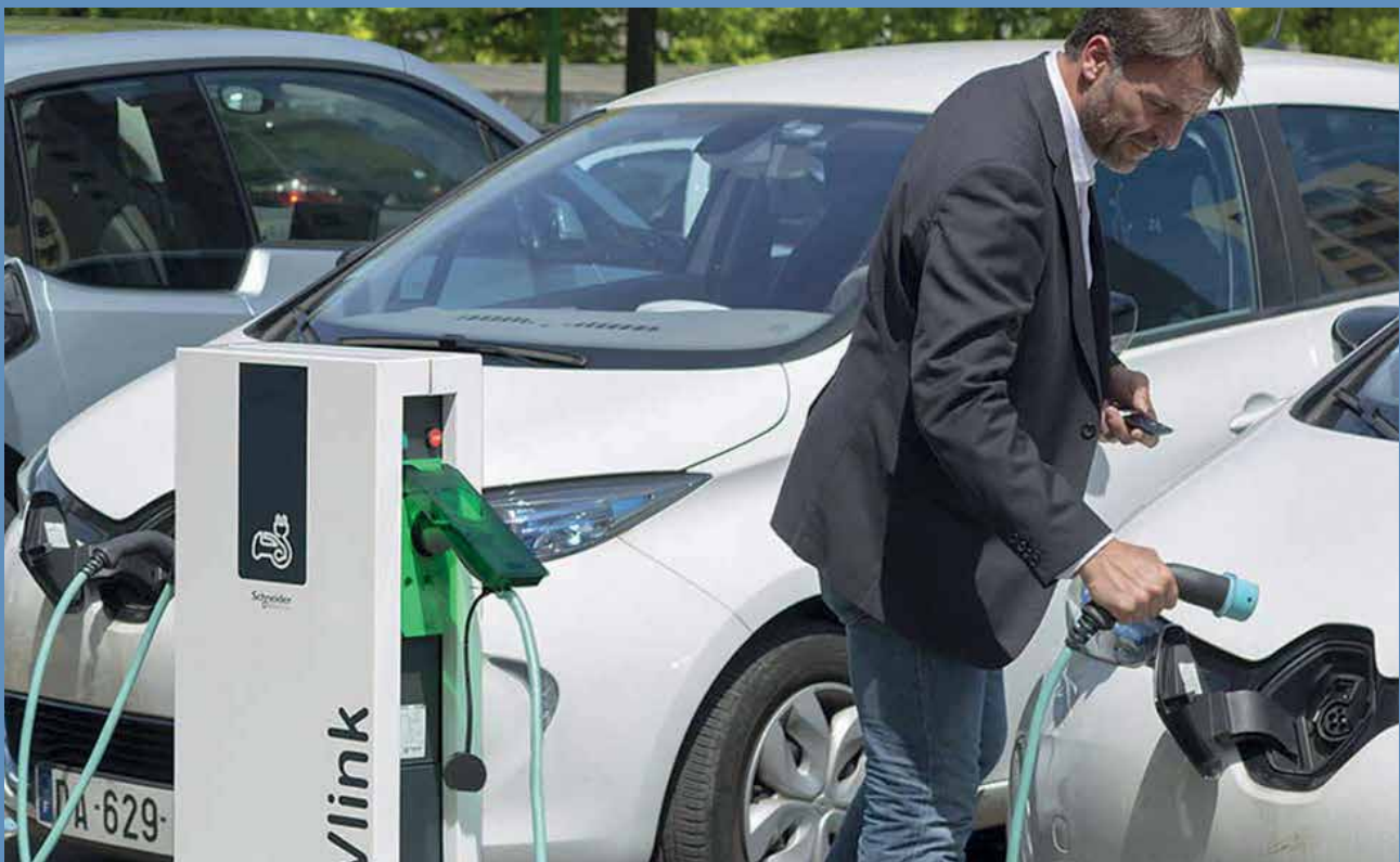
Figure 8. Dual socket public destination chargers.
