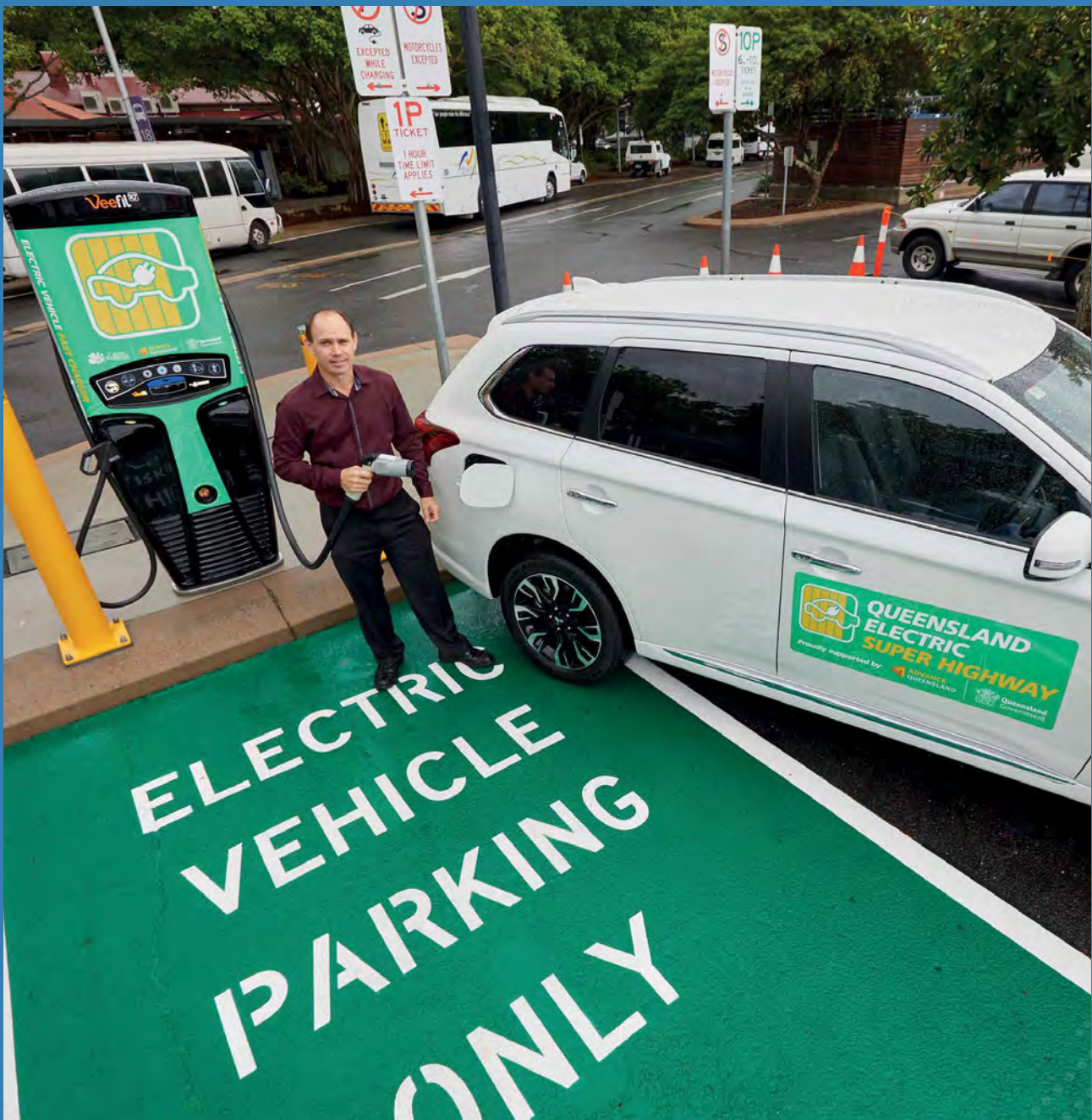
Figure 10. Cairns fast charging station on the Queensland Electric Super Highway
