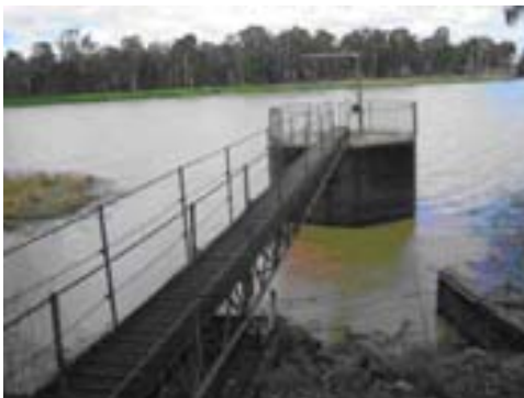
Photograph 1: Glenmore WTP intake structure on the Fitzroy River
