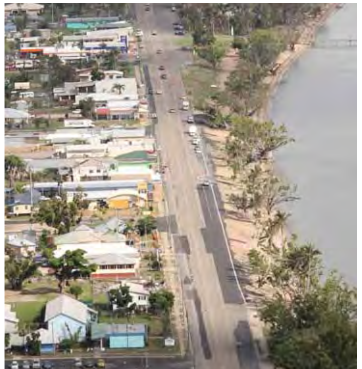
Photo 9 – Cardwell foreshore repaired after Cyclone Yasi.
