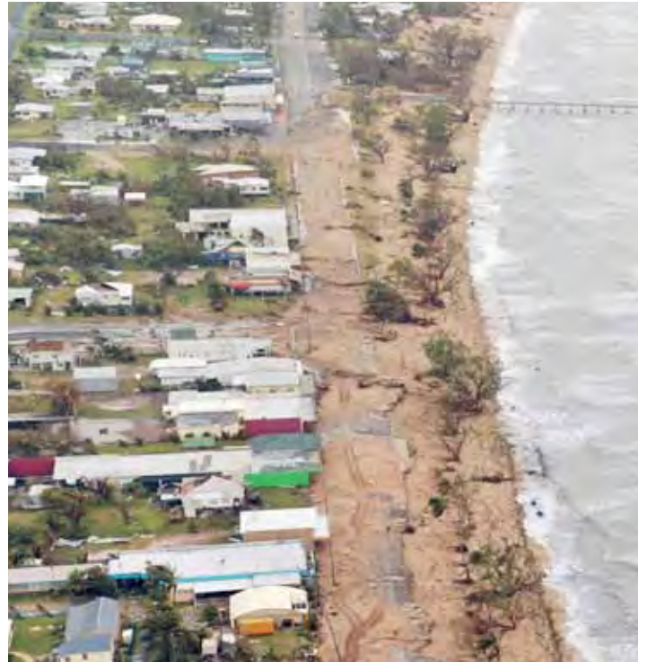
Photo 8 – Cardwell foreshore storm damaged after Cyclone Yasi.
