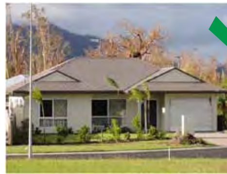
Photo 1 – roof has resisted loads near the design wind load in spite of minor debris damage and roller door failure
