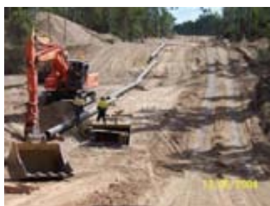
Photo ES-1: Clearing and Pipe Stringing
