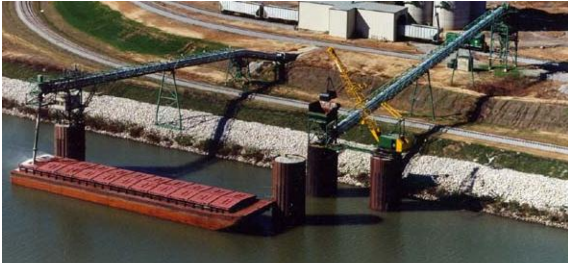
Photo 2.1: Example of a Barge Loading Facility
