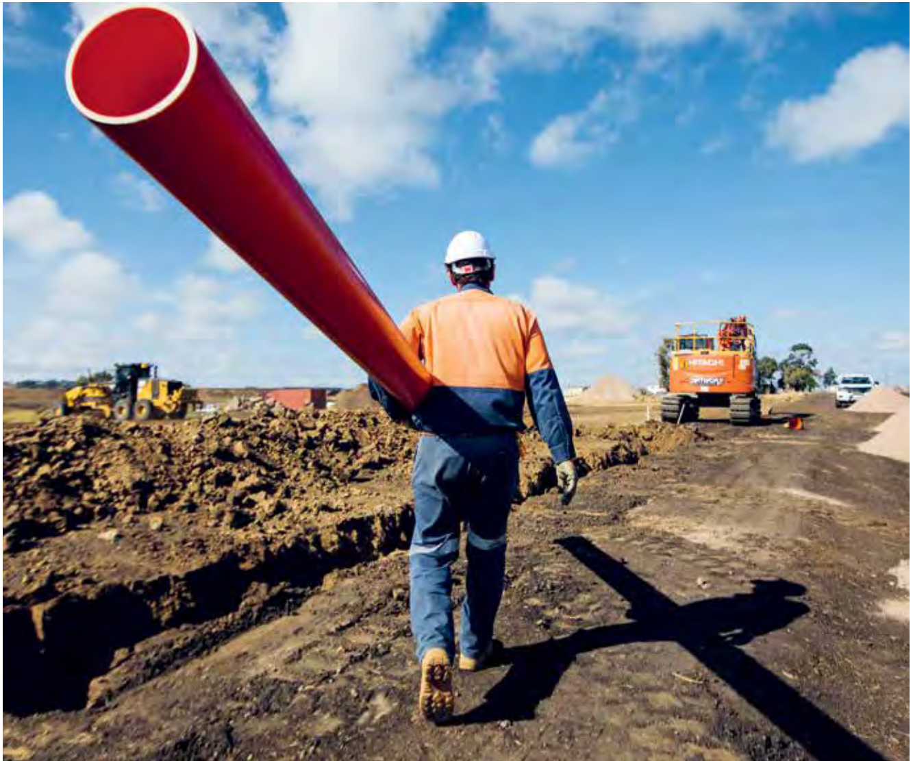
Construction of the Toowoomba Enterprise Hub, funded through Building our Regions
