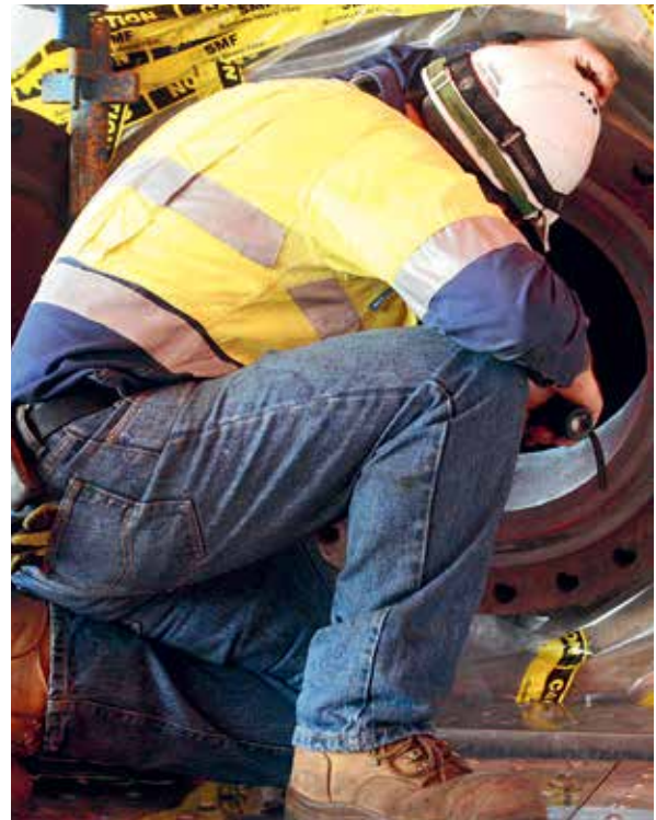
Stanwell Power Station unit overhaul
