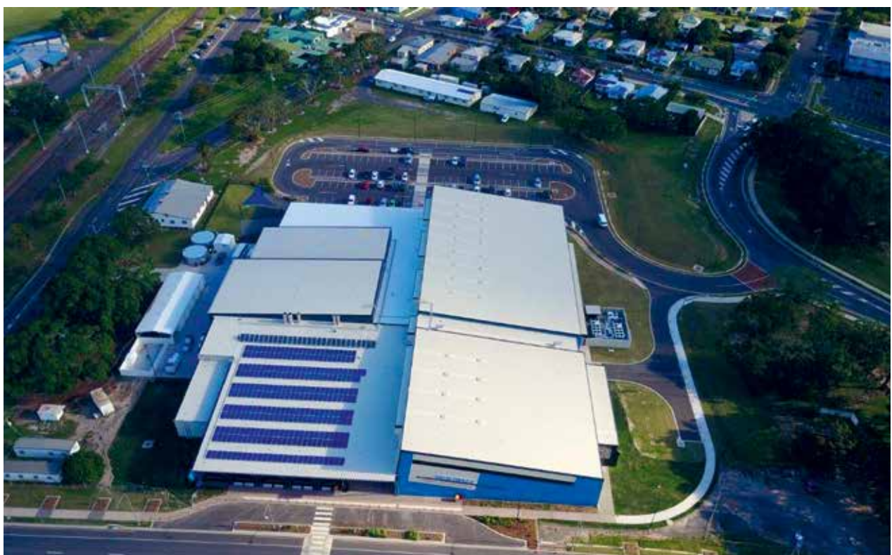
Bundaberg Multiplex Centre
