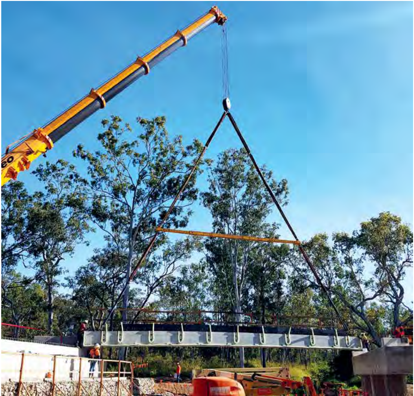
Peak Downs Highway structure replacement
