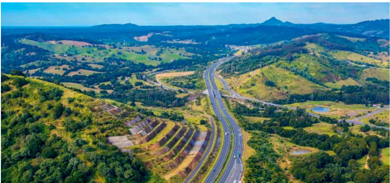
Bruce Highway upgrade – Cooroy to Curra
