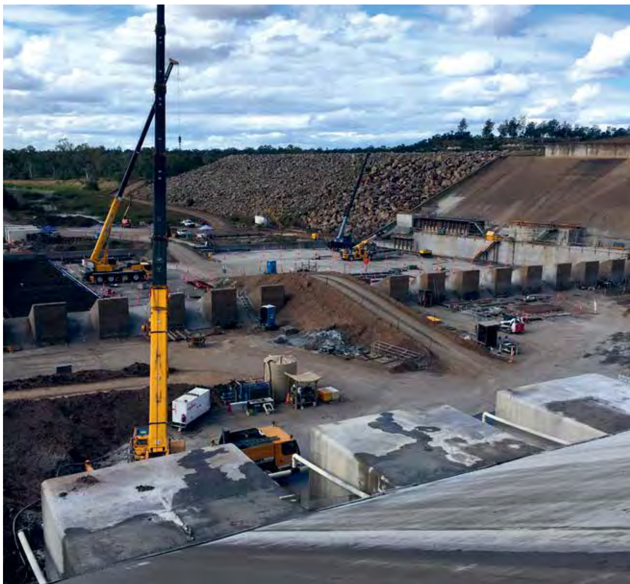
Fairbairn Dam improvement works
