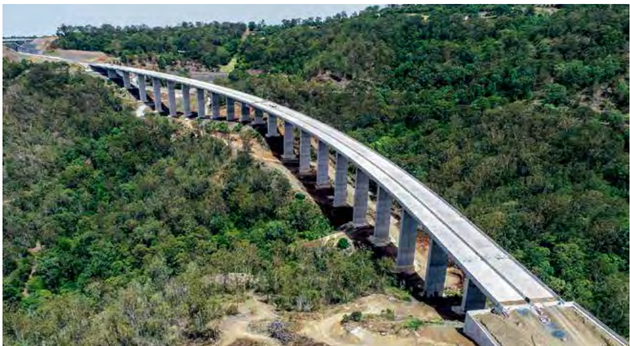
The viaduct along the Toowoomba Second Range Crossing
