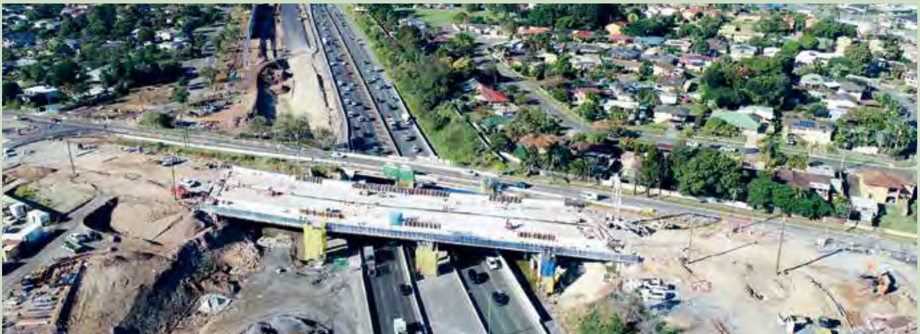
M1 Pacific Motorway Mudgeeraba to Varsity Lakes upgrade
