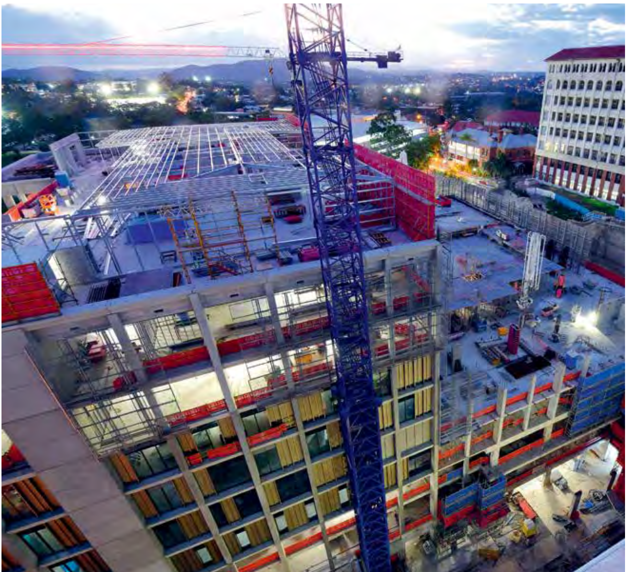
Construction of the Surgical, Treatment and Rehabilitation Services building at Herston
