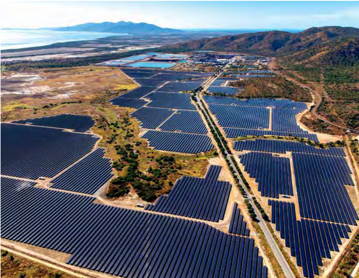
Sun Metals solar farm
