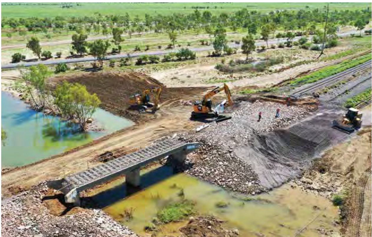
Mount Isa rail line recovery works
